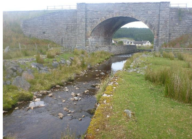
P1030804 – View downstream underneath railway bridge (NGR NH 786 322)
