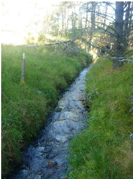
P1040023 – View towards the existing A9 culvert (upstream of the A9); the channel has been artificially straightened and bank/bed protected throughout (NGR NH 793 305)
