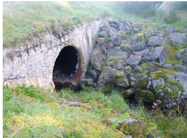
P1030994 – View of culvert underneath existing A9 (NGR NH 749 347)
