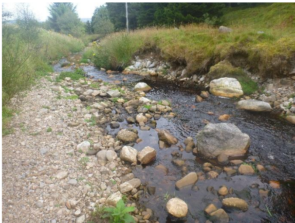
P1030760 – View downstream illustrating gravel/cobble bar opposite bank erosion (NGR NH 793 297)
