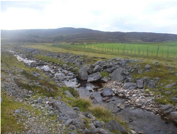
P1030800 – View upstream showing embankment on the left hand bank and stone protection throughout (NGR NH 784 321)
