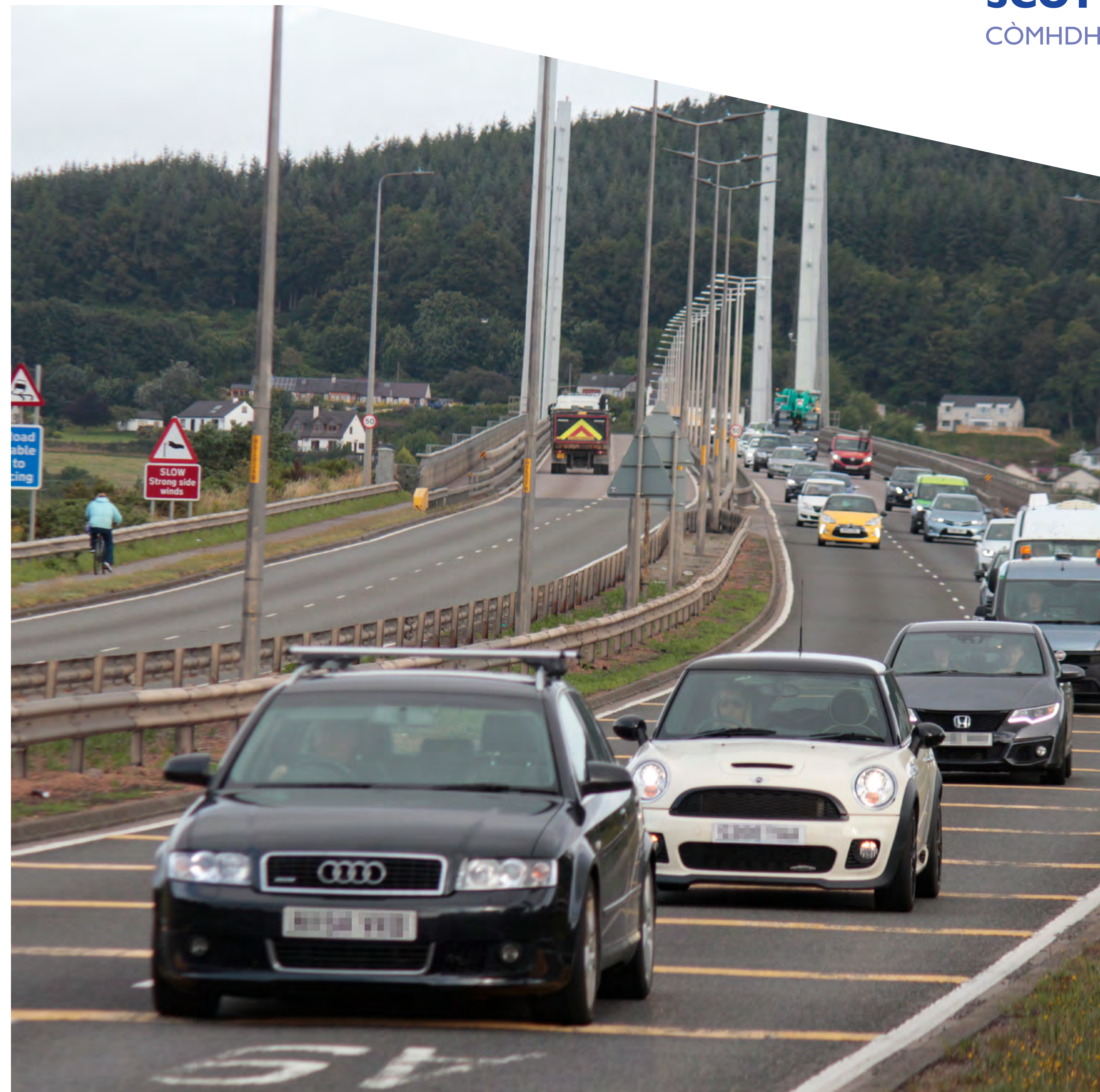
A9 looking north towards Kessock Bridge
