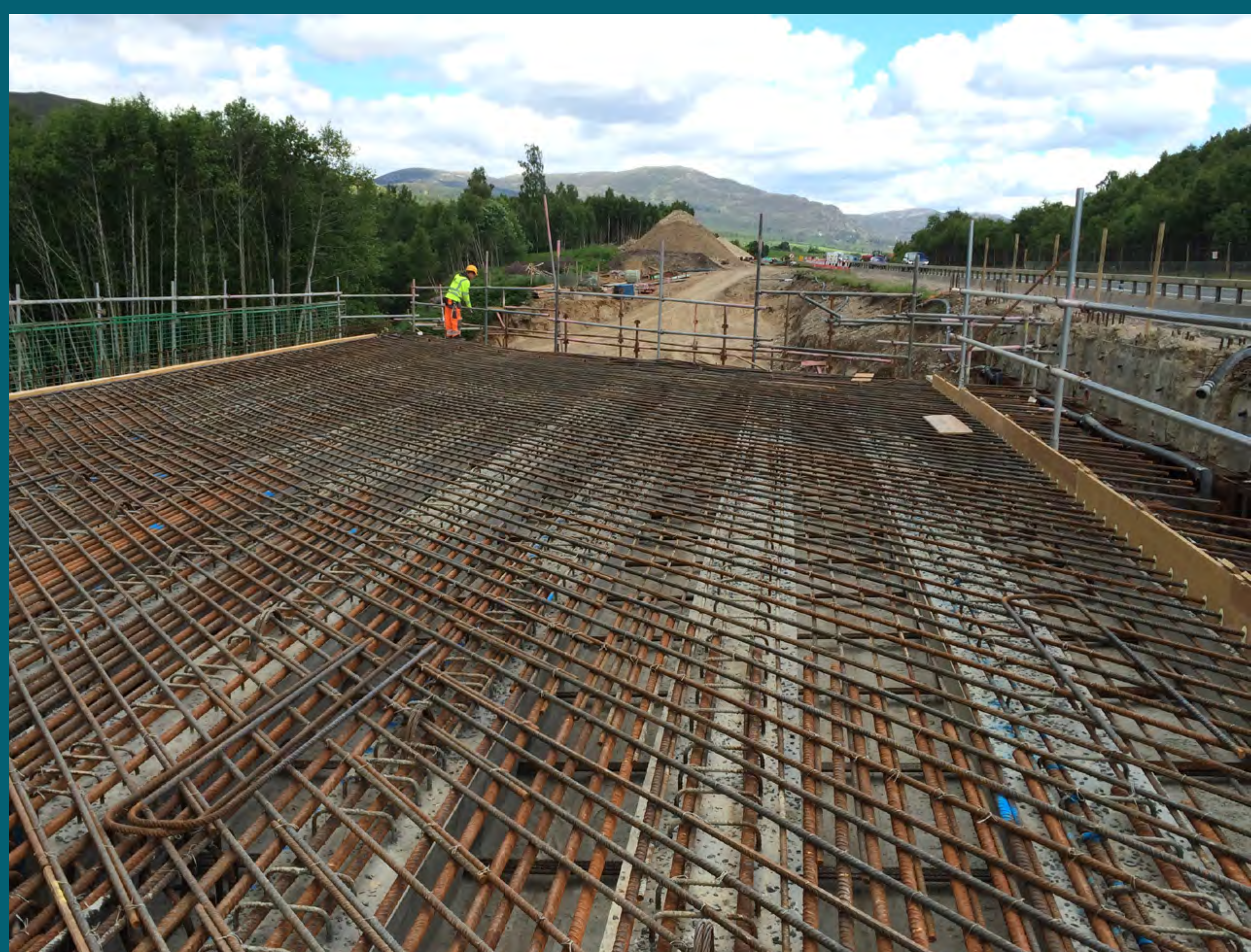
A9 Kincaig to Dalraddy – bridge deck
