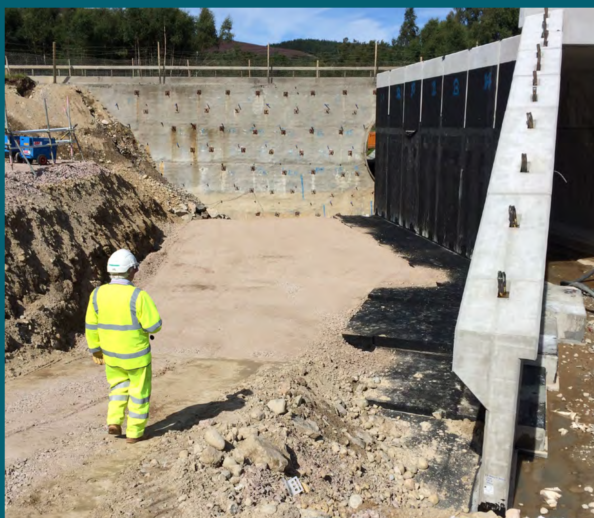
A9 Kincaig to Dalraddy – new culvert
