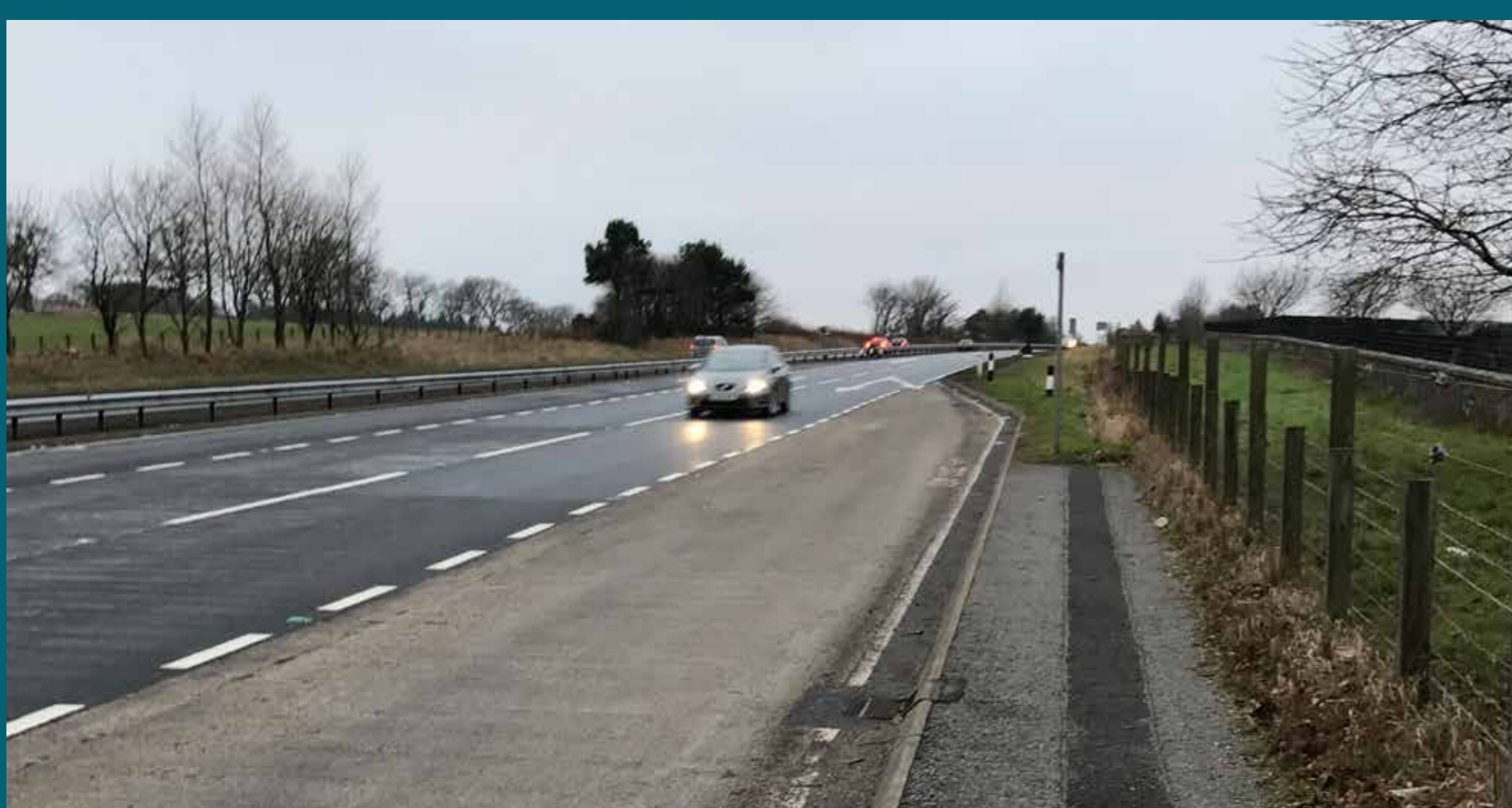
03 Footway adjacent to A90 northbound near centre junction
