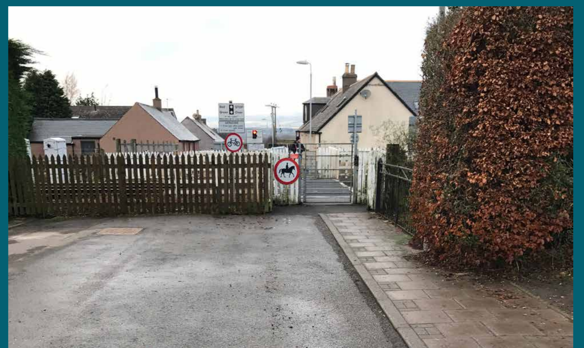
02 NMU railway crossing at Gardenston St
