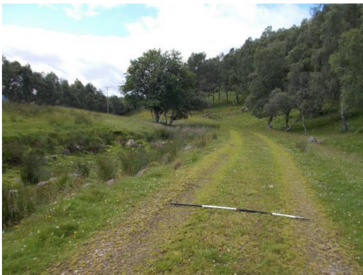
Photograph 4 (Section of General Wade's Military road, site 144)
