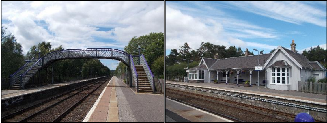
Photographs 12 & 13 Carrbridge Station (sites 190-193)
