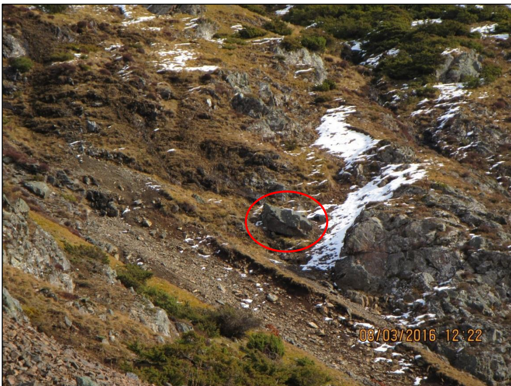
Figure 18 Erosion of the thin soil slopes at Slochd Mor. Note the large block which has failed from the crags above (circled)
