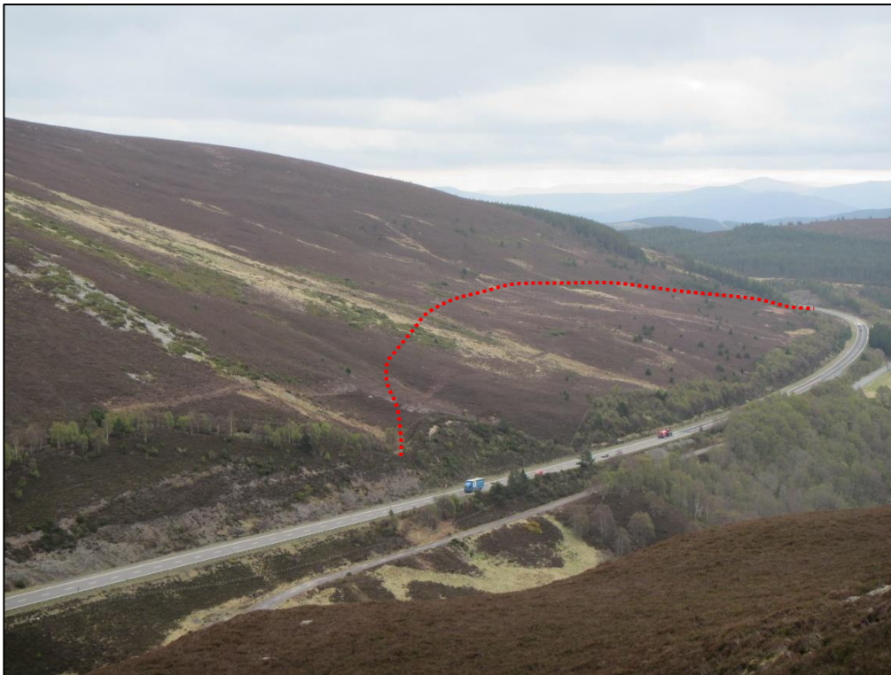
Figure 21 The approximate area where the depth to rockhead is currently uncertain. The extents are indicative only.
