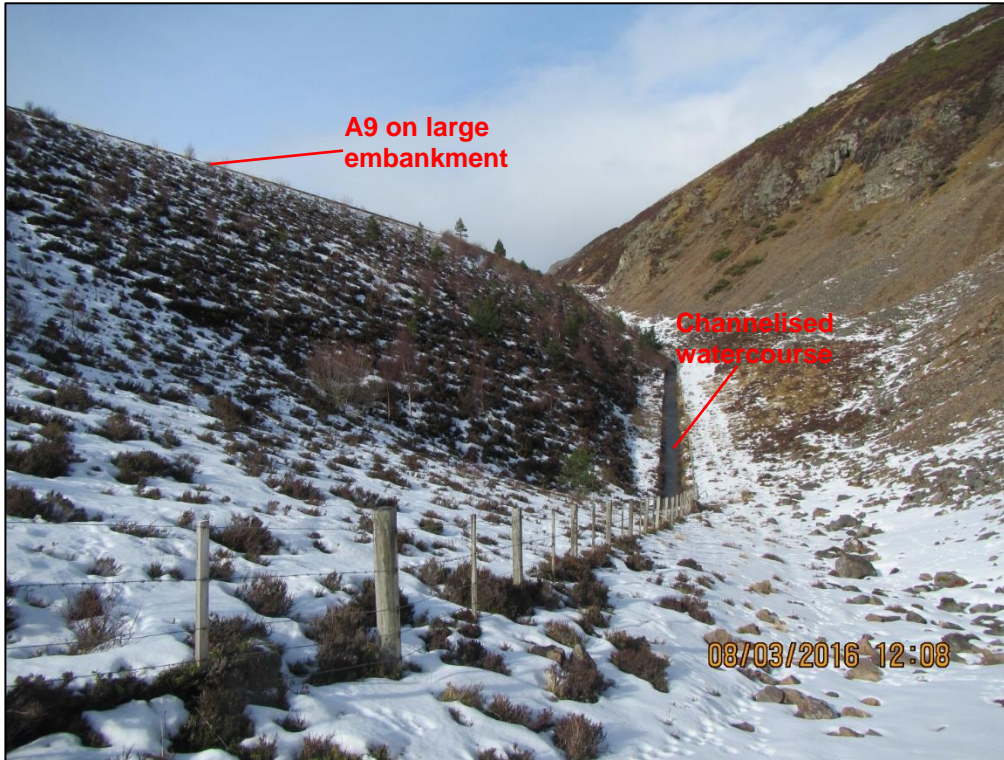
Figure 5 View to the northwest of the glacial hollow at Slochd Mor and the embankment that the A9 is carried upon.
