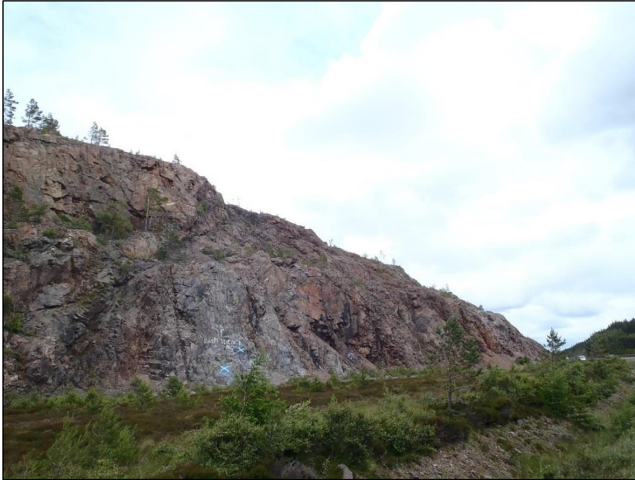
Figure 15 Existing Slochd Beag rock cutting formed in the late 1970s / early 1980s during construction of the A9
