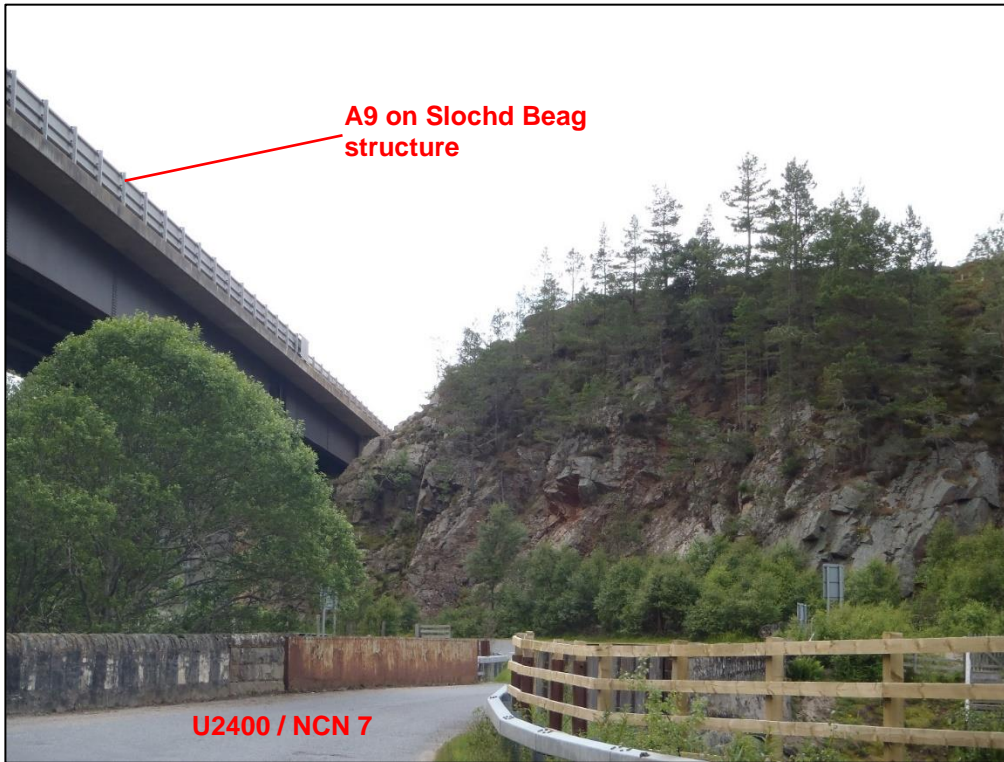
Figure 3 View to the west of the U2400 bridge over the Highland Main Line with the A9 above.
