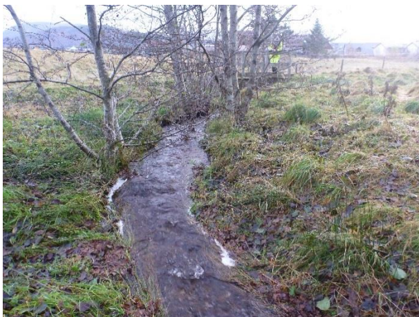
P1040853 – View immediately downstream of A9 culvert outlet (NGR 2895 8141)
