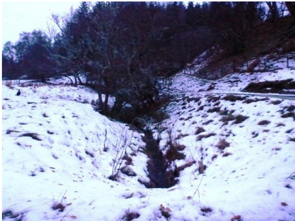
P1040486 – View upstream from track crossing; track shown on the right (LHB) (NGR 2870 8103)
