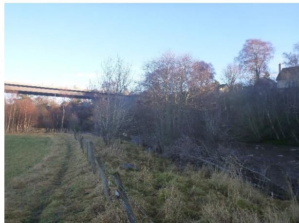
P1040609 – View downstream towards existing A9 bridge over the Dulnain (NGR 2856 8225)
