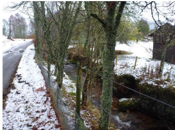
P1040449 – View downstream towards existing A9 crossing; the channel here has been channelised and bank protected around residential properties (NGR 2881 8107)
