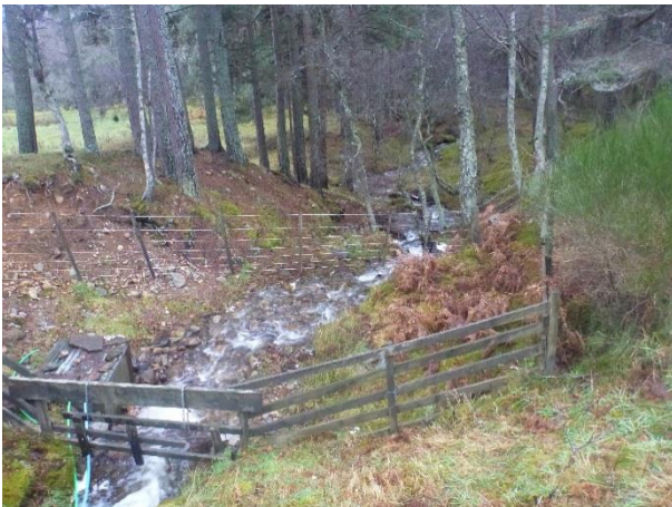
P1040798 – View from existing A9 crossing downstream (NGR 2902 8164)
