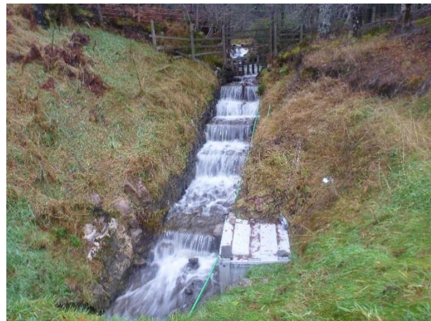
P1040794 – Artificial concrete steps leading into existing A9 crossing (NGR 2902 8164)
