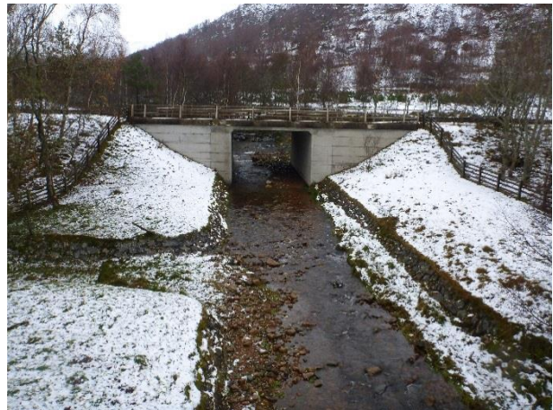
P1040470 – View upstream towards A9 crossing (NGR 2884 8106)
