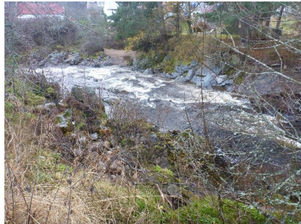
P1040945 – Bedrock channel leading into Carrbridge (NGR 2906 8230)
