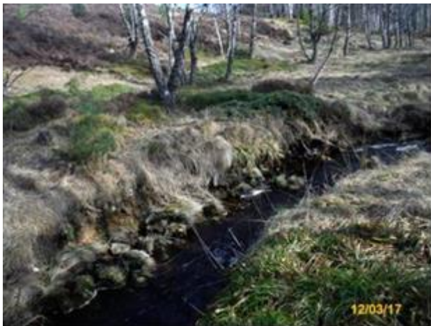
Figure 14-19 Erosion on bend downstream of railway bridge
