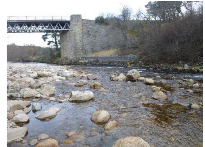
Photo P10107 Downstream of A9
