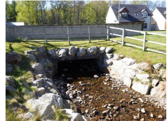
Photo P1010818 Upstream of A9
