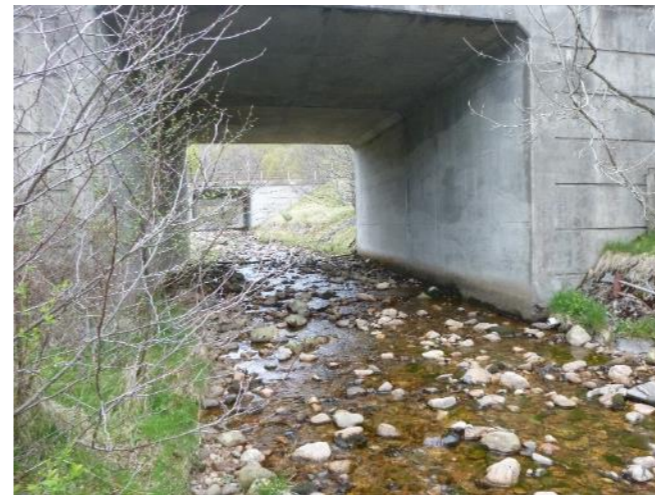
Photo P1010939 A9/A95 Crossing (Looking Upstream)
