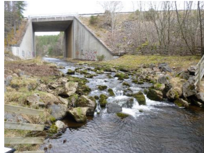
Photo P1010744 A9 Crossing (Looking Upstream)
