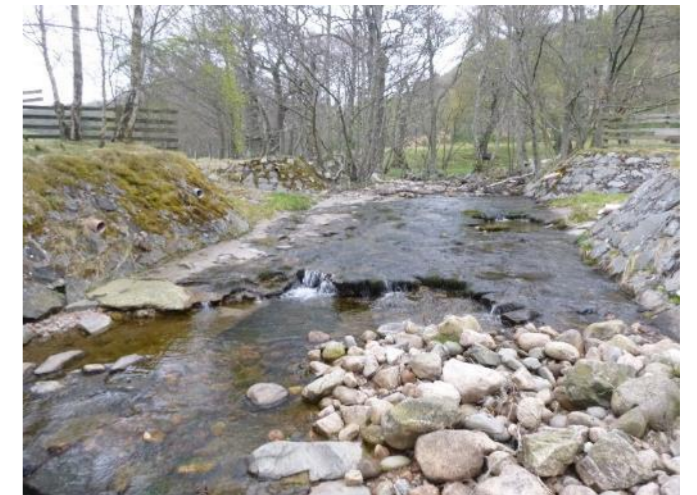
Photo P1010945 Upstream of A9
