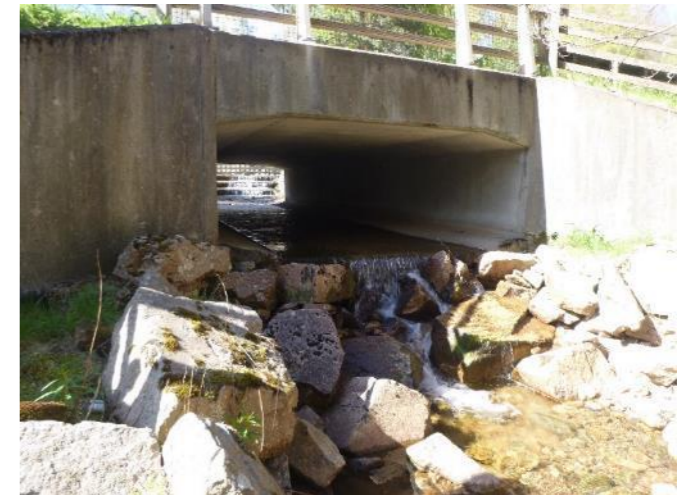
Photo P1010893 A9 Crossing (Looking Upstream)
