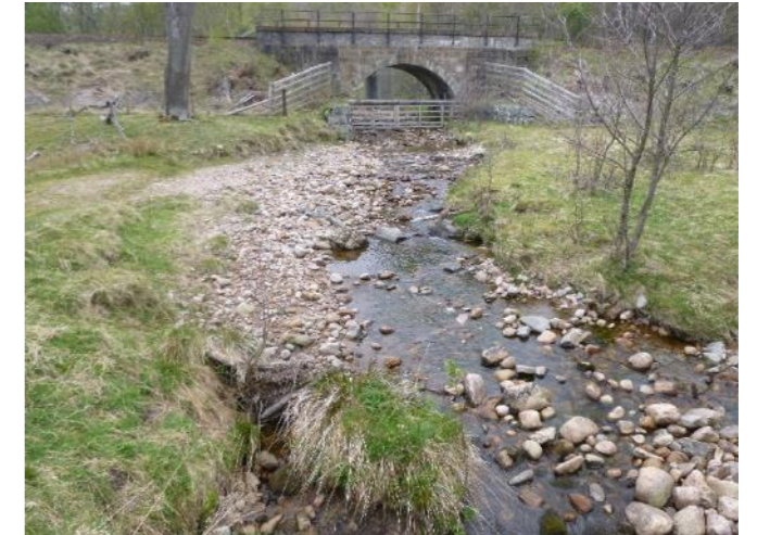
Photo P1010936 Downstream of A9
