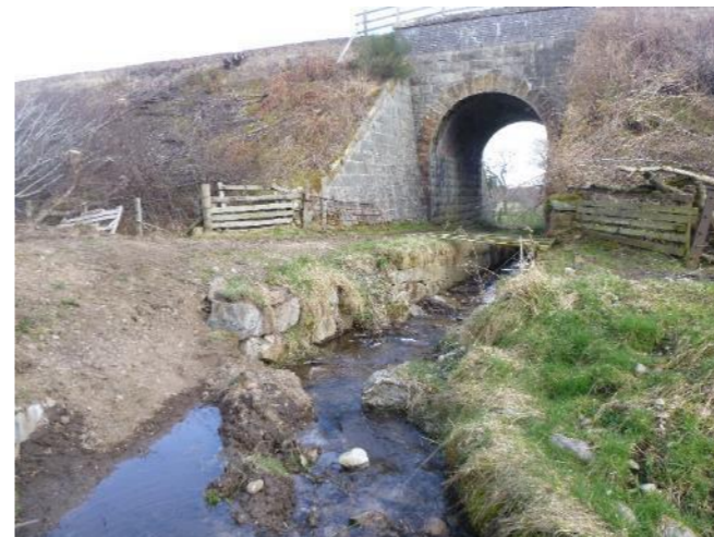
Photo P1010730 Downstream A9 Showing Rail Bridge
