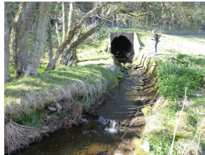
Photo P1010912 A9 Crossing (Looking Upstream)
