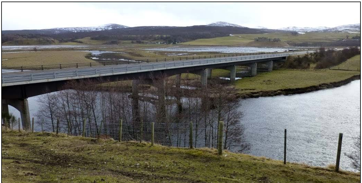
Photograph 3-1: River Spey Bridge at Kingussie/ Insh Marshes
