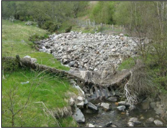
A) Large volume of deposited materials upstream of A9 crossing B) Out-of-bank flow and deposition of material downstream of A9
