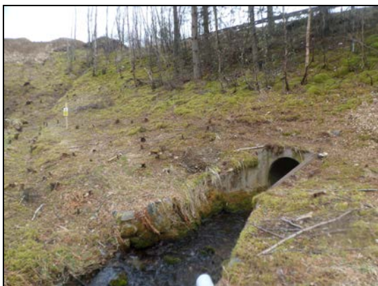
A) Upstream of A9 crossing (looking south)
