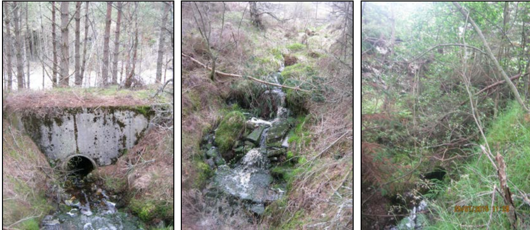
A) Upstream looking towards A9
