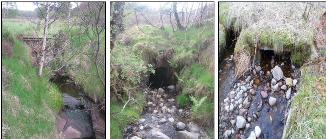
A) Metal sluice upstream of A9
