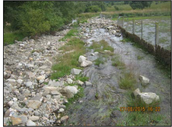
A) Large volume of deposited materials upstream of A9 crossing B) Out-of-bank flow and deposition of material downstream of A9
