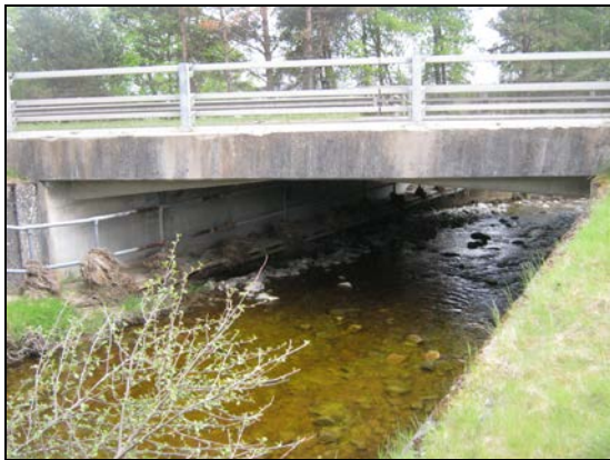
A) Upstream of A9 crossing (looking south)
