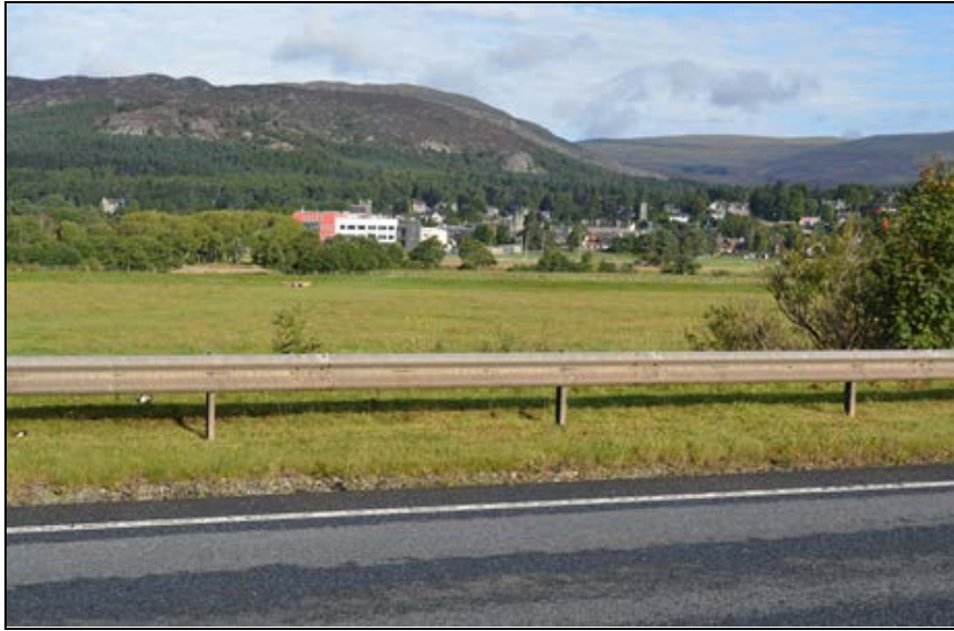
Photograph 13:9: View west towards Kingussie from existing Lay-by 114
