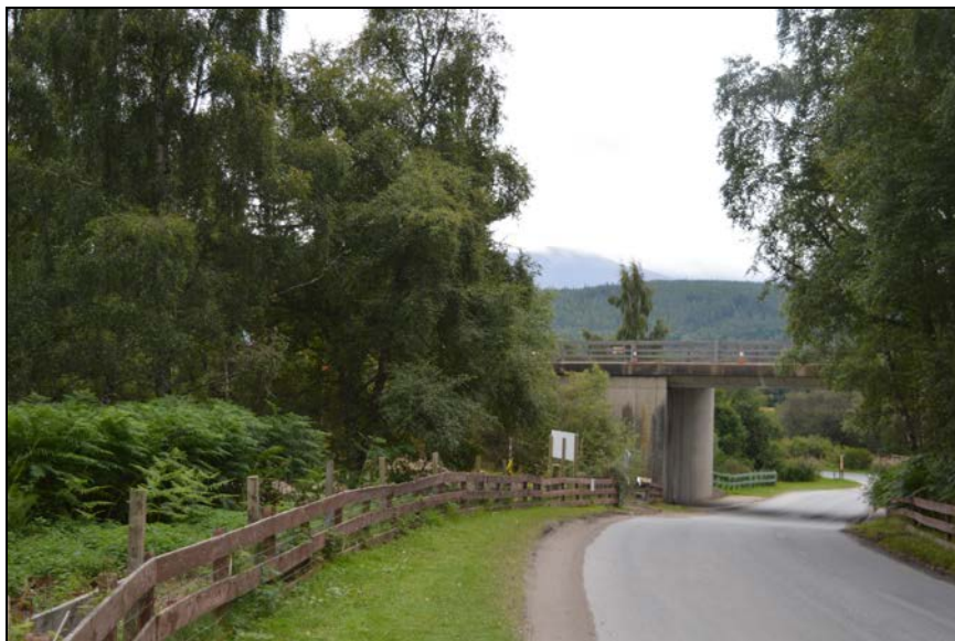
Photograph 13:13: View east to A9 bridge from Highland Wildlife Park access road
