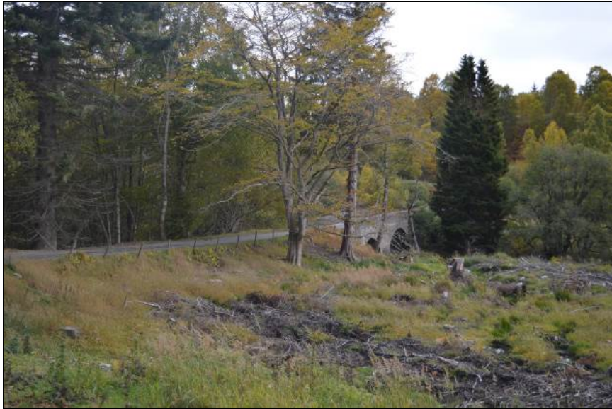
Photograph 14-1: NCN7 adjacent to the A9 on road to Invernahavon
