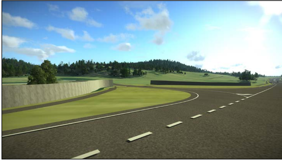
Figure 14-8: Indicative view of left-in left-out access at Balavil Mains with noise mitigation barriers
