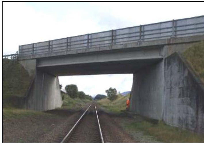
Photograph 4-2: Existing Kingussie rail bridge
