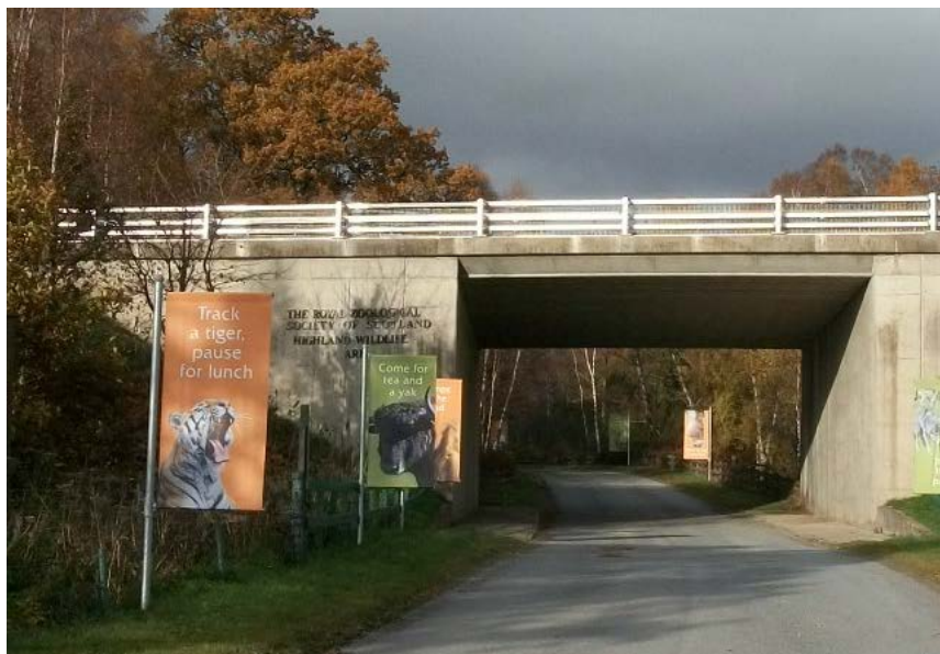
Photograph 4-3: Existing Wildlife Park bridge
