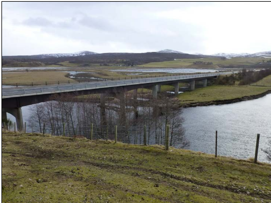
Photograph 4-1: Existing River Spey bridge
