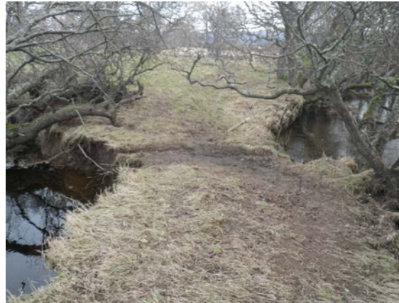
Photograph 23: Looking east, area of scour to left, Spey to right. Bank is not breached
