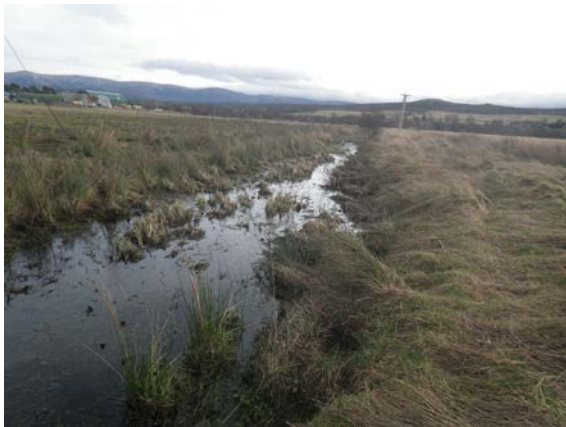
Photograph 55: Downstream low embankment on right bank side
