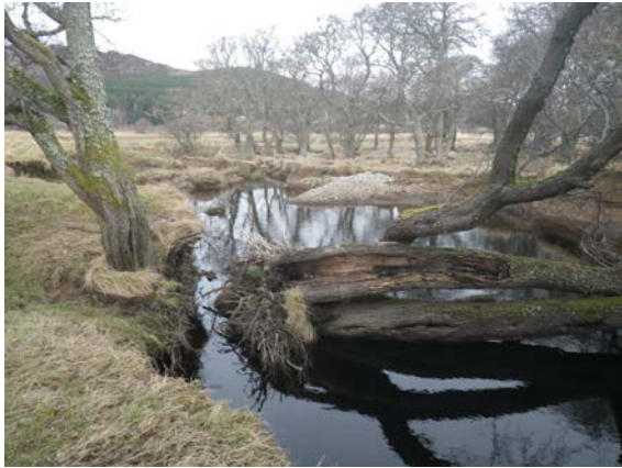
Photograph 22: Looking north, area of scour through embankment, uprooting trees
