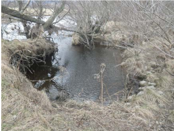
Photograph 19: Breach in embankment
