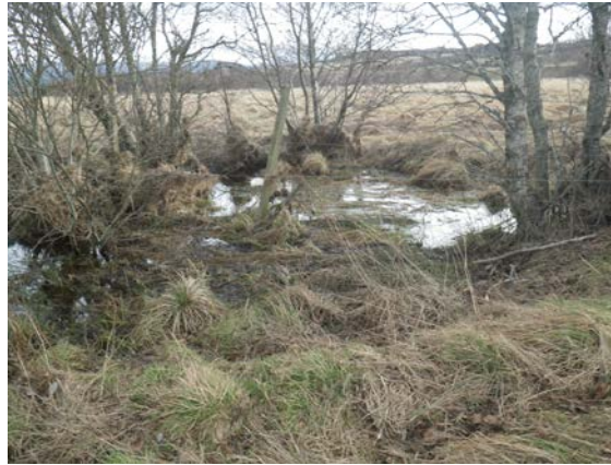
Photograph 2: Ponding in lower wider section of ditch
