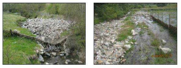
A) Large volume of deposited materials upstream of A9 crossing B) Out-of-bank flow and deposition of material downstream of A9
