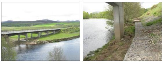
A) Looking towards Spey crossing from north embankment B) Existing erosion protection on left bank of Spey
