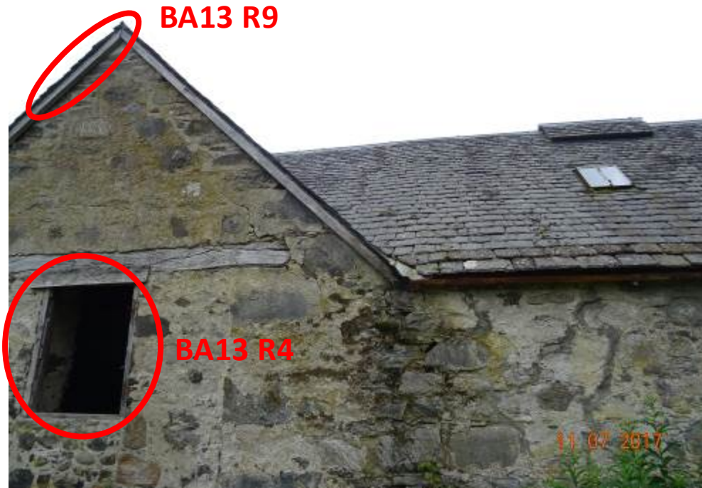
Photograph 12.8.22: Balavil BA13 roosts northern side of building
