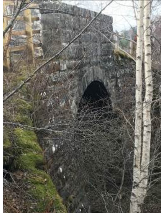
Photograph 12.8.13: North side of railway bridge
