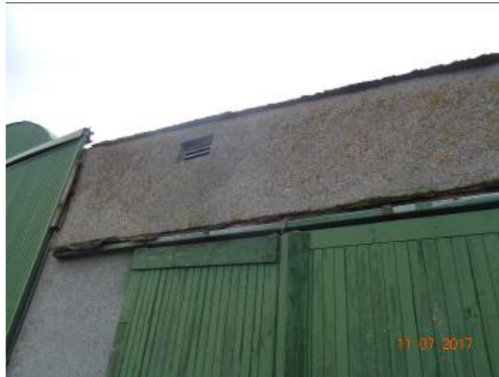
Photograph 12.8.11: Barn opposite Kerrow Cottage
