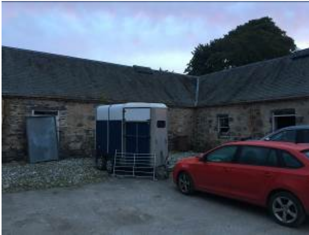
Photograph 12.8.6: Balavil BA13 courtyard
