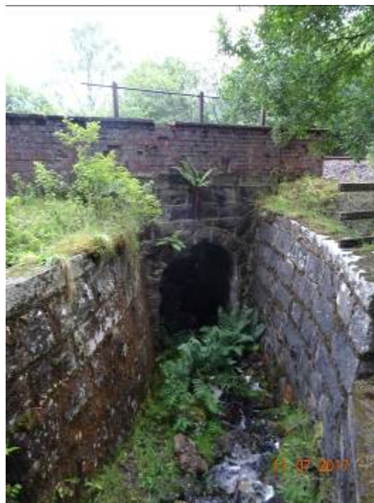
Photograph 12.8.3: Livestock tunnel BA1
