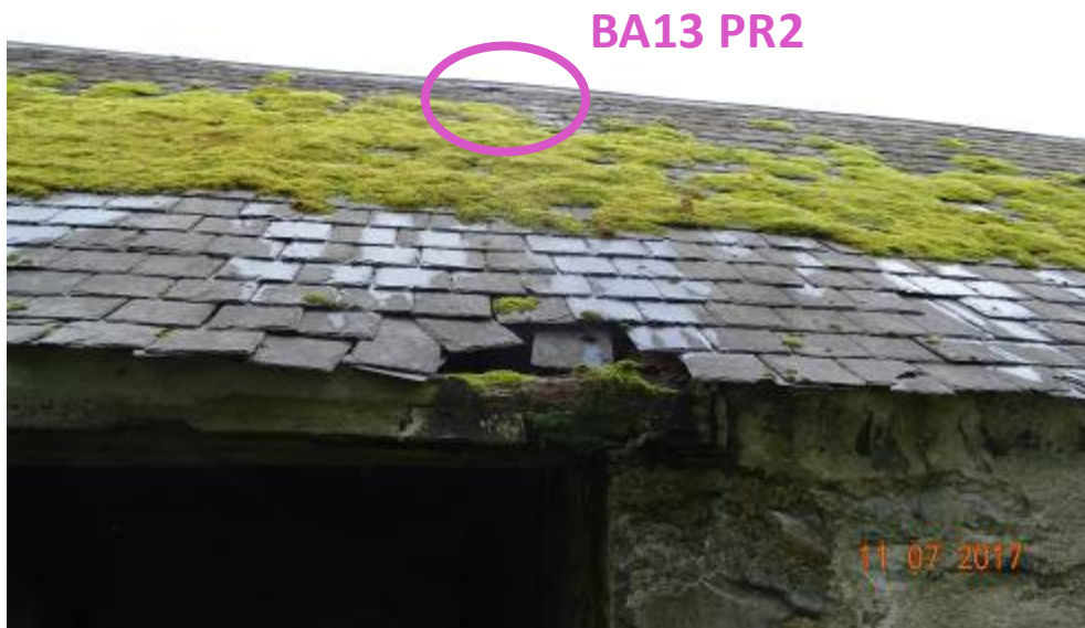
Photograph 12.8.23: Balavil BA13 roosts separate eastern structure
