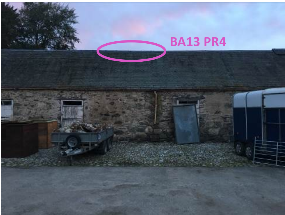
Photograph 12.8.19: Balavil BA13 roosts northern courtyard
