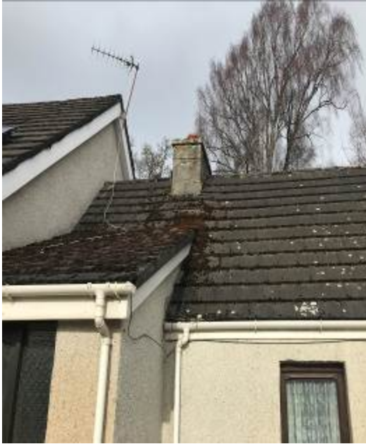
Photograph 12.8.14: Roof tiles, chimney, roughcast walls in good condition
