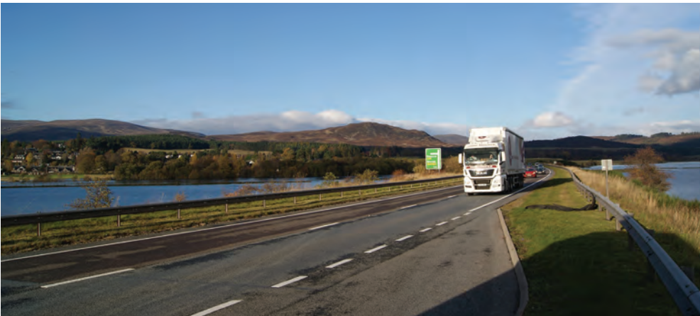
Photograph 3-5: Flood waters visible adjacent to approach to River Spey crossing
