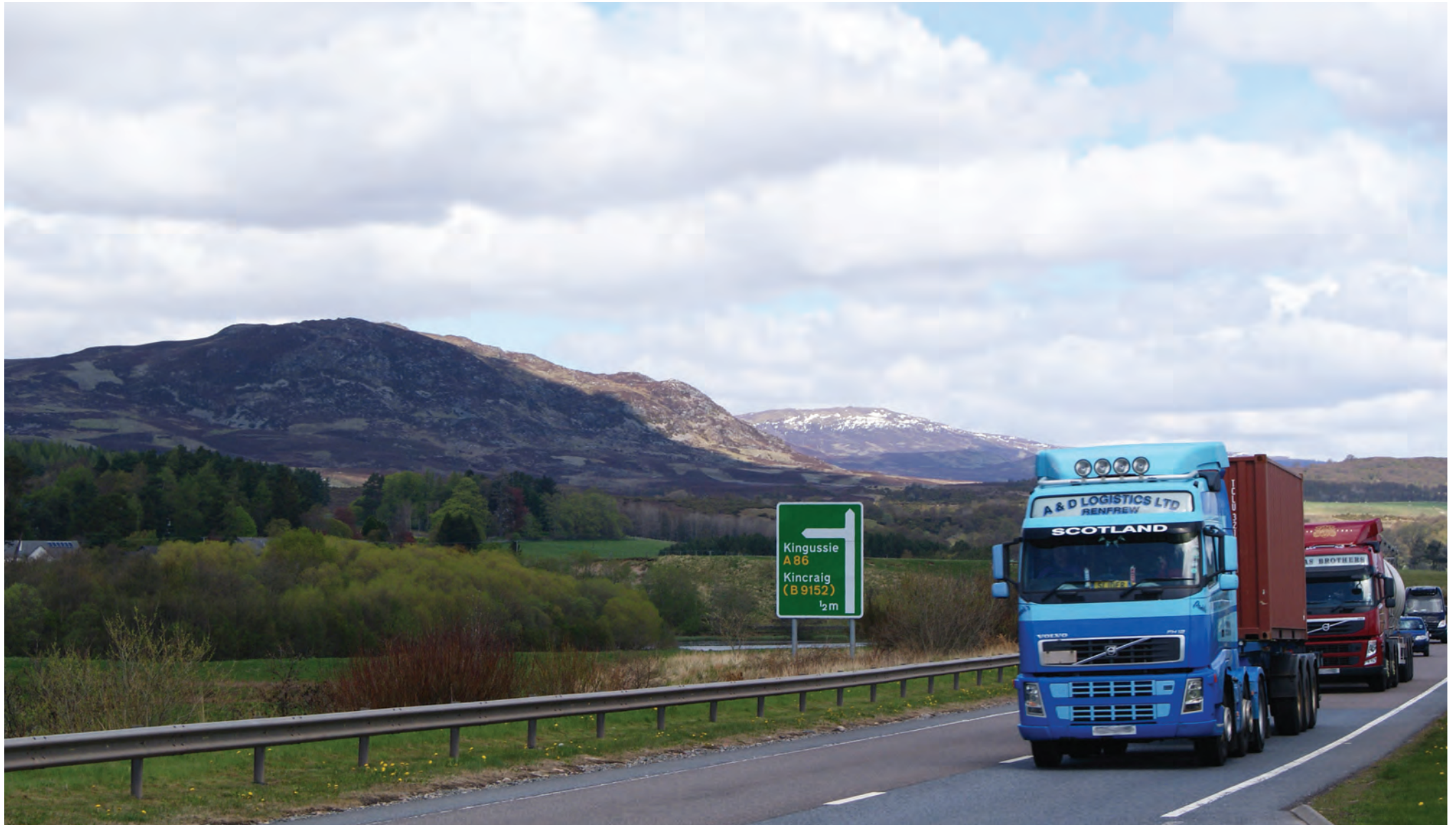
A9 looking northwest towards Kingussie
