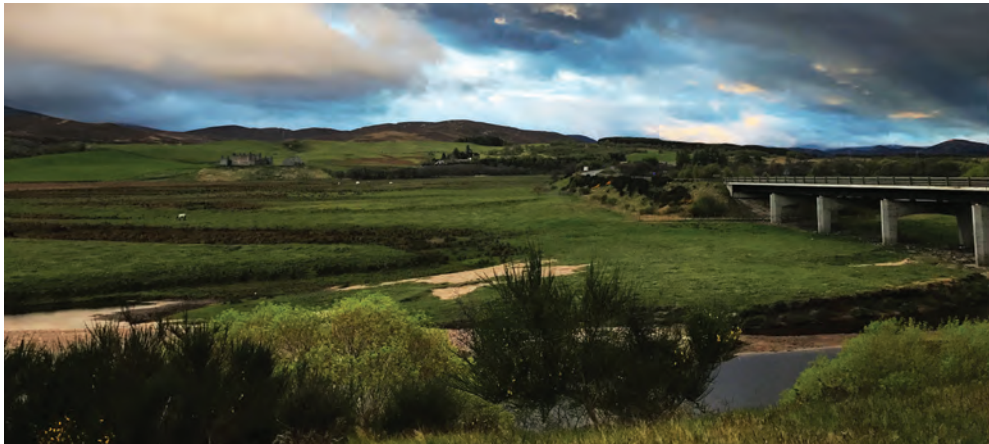
Photograph 3-7: Existing A9 River Spey crossing at Insh Marshes NNR
