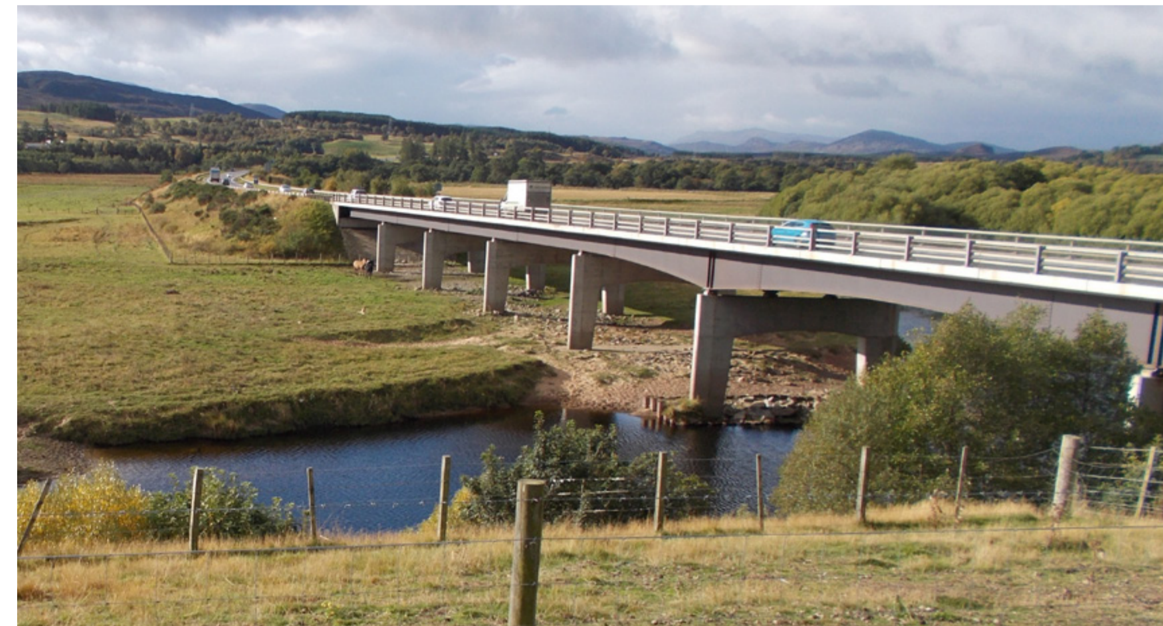
Existing River Spey bridge, Kingussie
