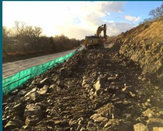
Example of KinCraig roadworks under construction
