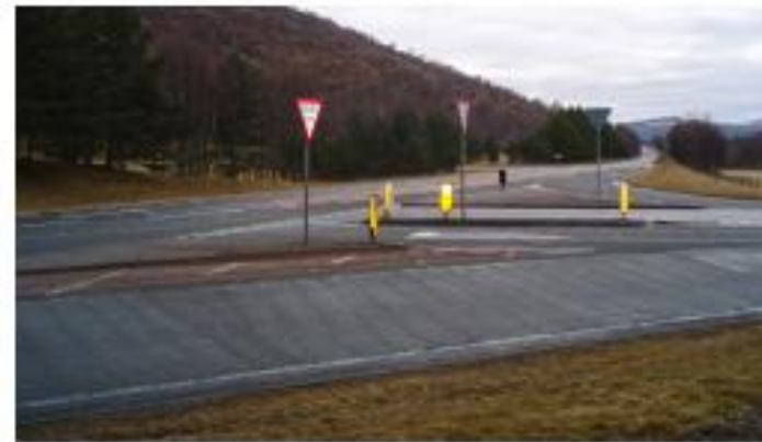
Existing Aviemore South junction
