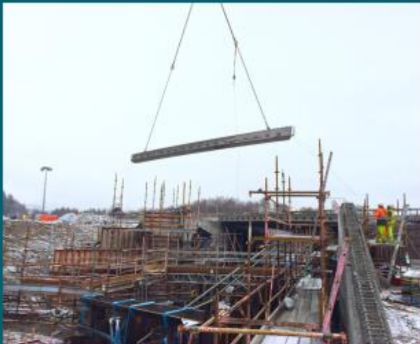
Example of KinCraig underpass under construction
