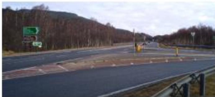
Existing Granish junction
