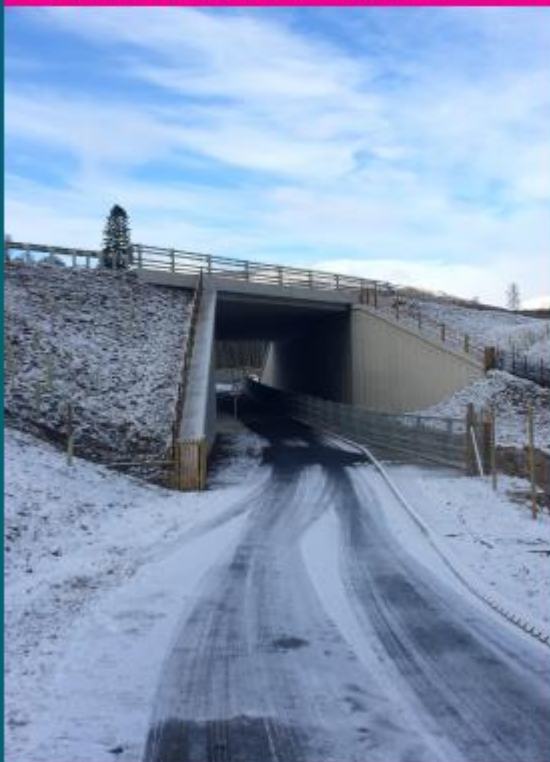
Example of Kincaig underpass (completed)
