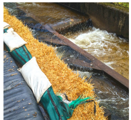
The self-built filtration device mostly used materials already found on the site
