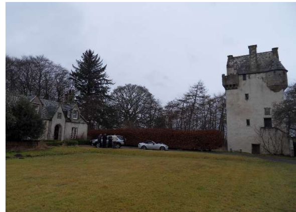
Photograph 16.4: Coxton Tower House (MMS163 left) and Coxton Tower (MMS164 right)
