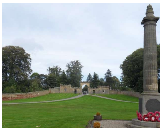
Photograph 16.6: Looking north-east towards the Gordon Castle West Lodge MMS092
