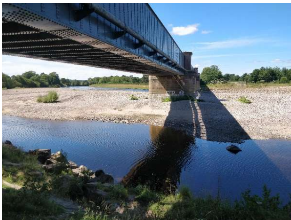
Photograph 20.1: River Findhorn – downstream face of the Viaduct
