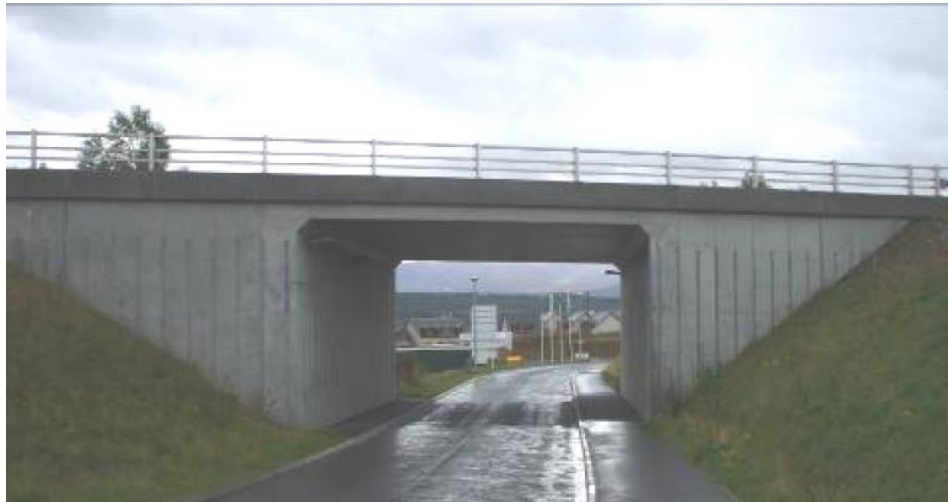
Photograph 2.11.8 High Burnside Underpass
