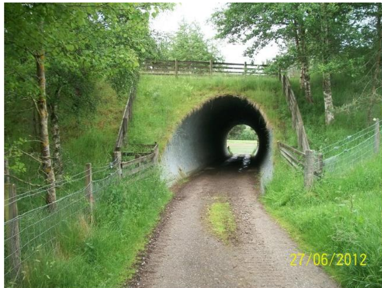
Photograph 2.11.2 Ballinluig pedestrian underpass
