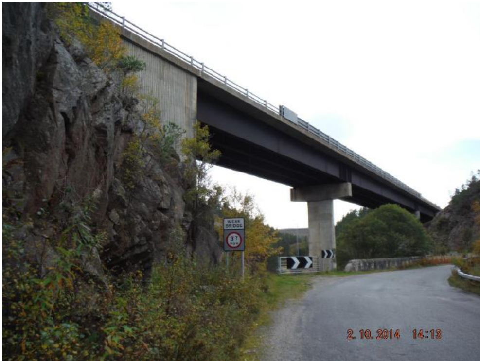
Photograph 2.11.13 Slochd Beag Bridge
