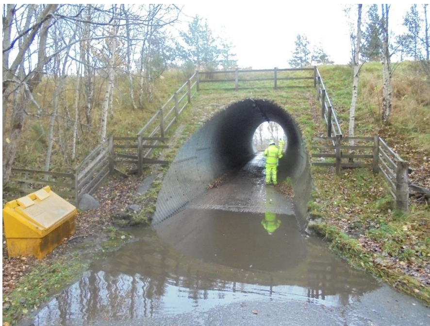
Photograph 2.11.5 Craig Dhu Underpass
