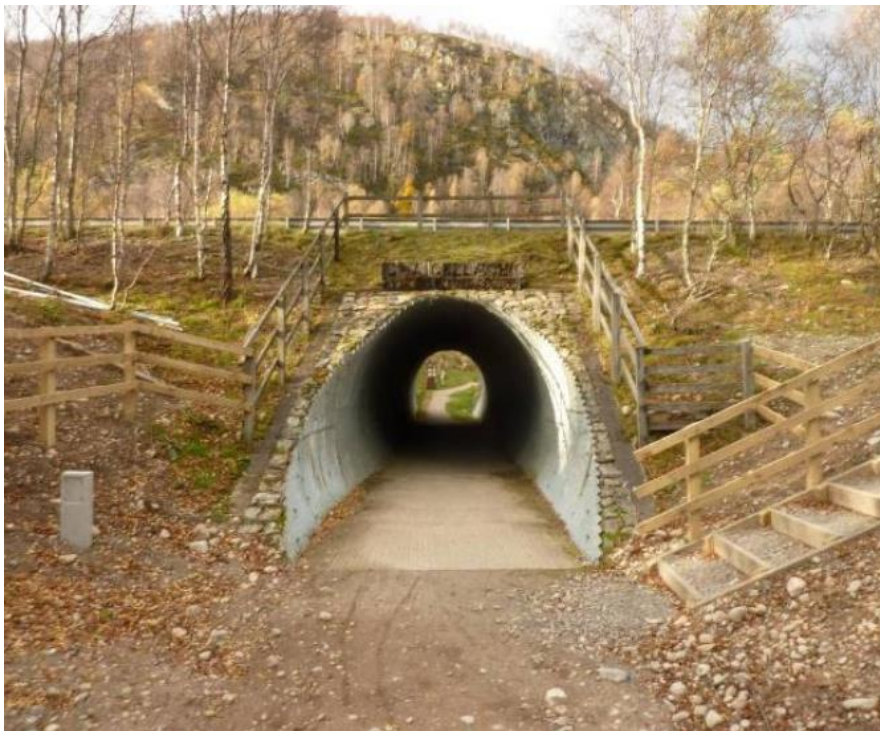
Photograph 2.11.6 Craigellachie Nature Reserve Underpass
