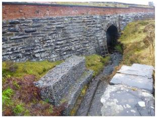
P1040970 – Channel between the railway and A9 was lined with gabion and stone wall protection through two culverts (NGR 2837 8254)
