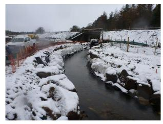
P1040416 – View upstream towards existing A9 crossing; the channel had been lined artificially with rip-rap and boulder protection as part of the ongoing construction works (NGR 2855 8092)
