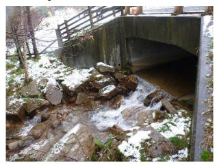
P1040425 – View of culvert outlet with signs of incision downstream and the invert was perched above the channel bed (NGR 2857 8095)
