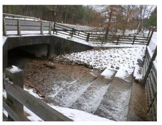
P1040419 – View of existing A9 crossing with concrete stepped cascade leading into culvert (NGR 2857 8095)
