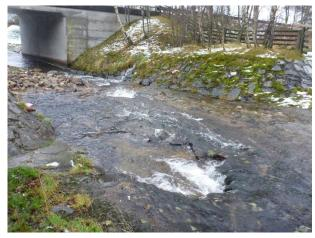
P1040468 – Collapse concrete/cobble bed leading towards the existing A9 crossing (NGR 2884 8106)
