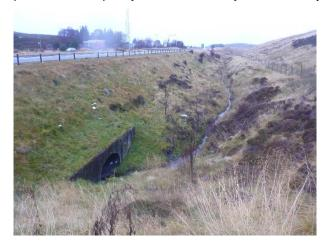
P1040955 – The channel has been realigned and constrained into a narrow artificial valley through a series of culverts (NGR 2836 8256)
