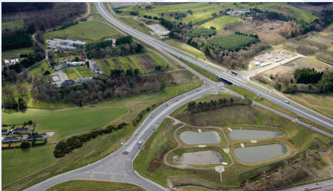
Road users on the new trunk road
