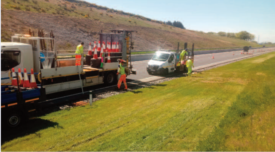
Traffic management being removed following grass cutting operations
