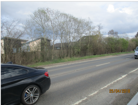
Existing A96 looking towards adjacent properties
