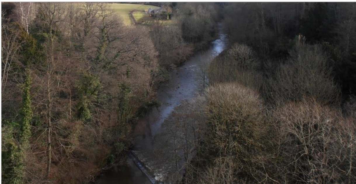
Plate 11-1 Downstream View of the River North Esk from the A7 Road Bridge
