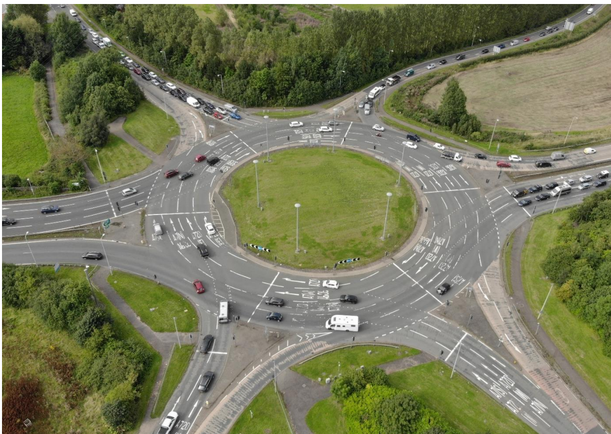
Plate 14-1 View of the Existing Roundabout looking North
