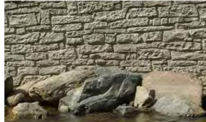
Fig. 20 Formwork liners can create various patterns within in-situ concrete (Max Frank)
