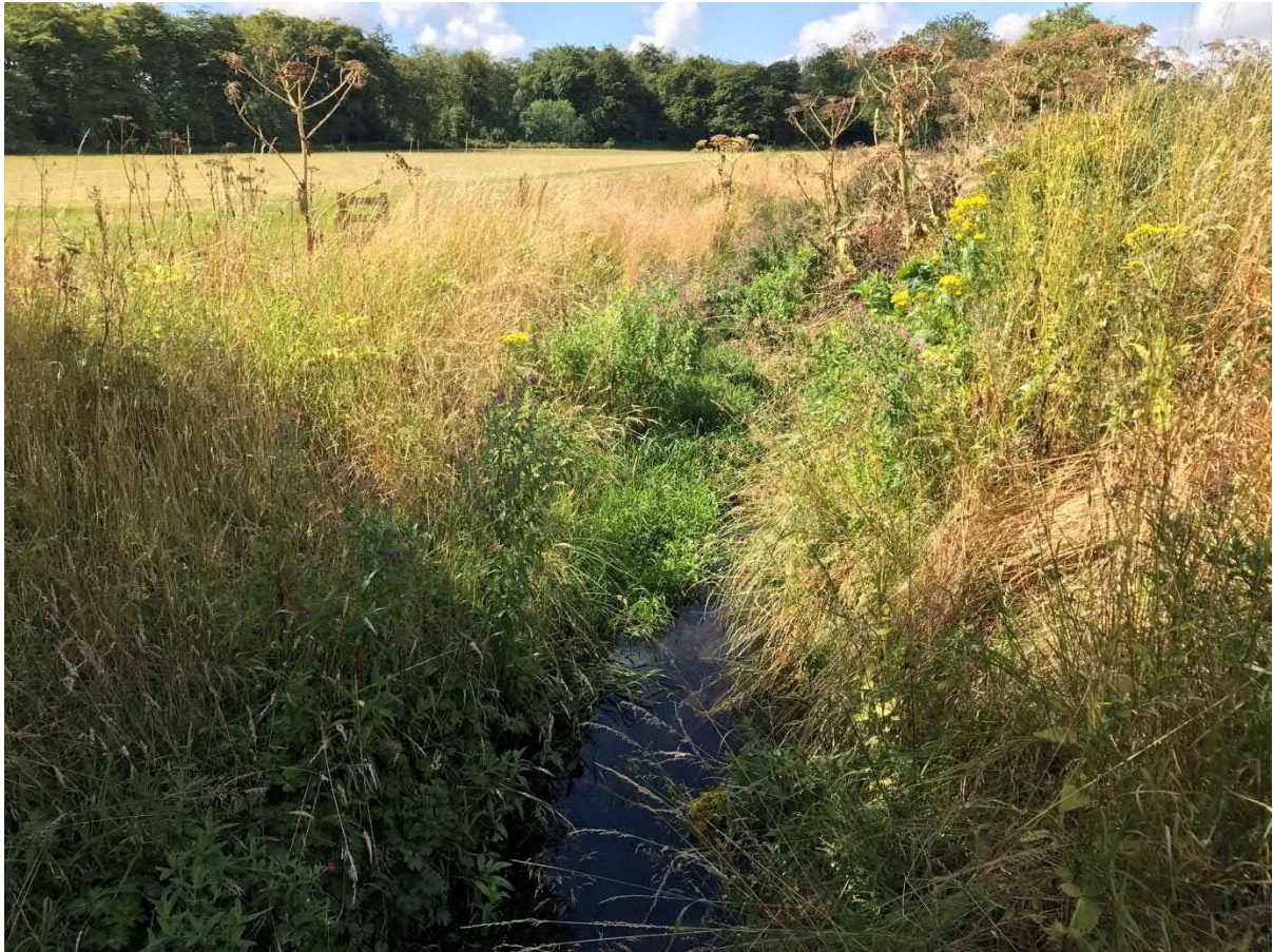
Photograph 3: Area upstream of A7 culvert
