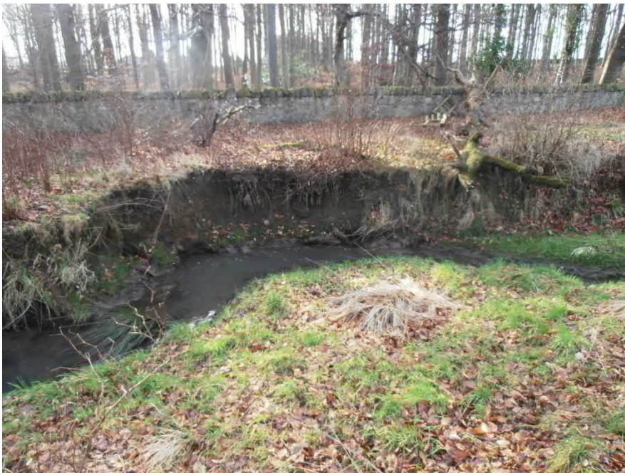
Figure 3 Erosion of bank upstream of pond and fine sediment berm formation
