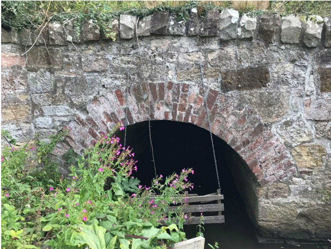
Photograph 7: Inlet of Old Dalkeith Road culvert
