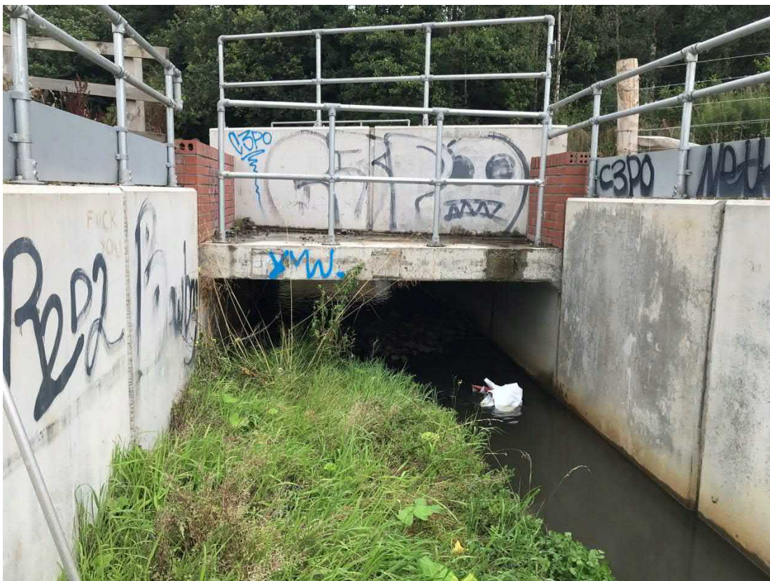
Photograph 8: Culvert leading into Dalkeith Country Park
