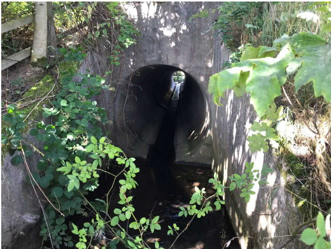
Photograph 6: A7 culvert outlet
