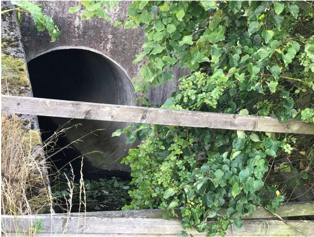
Photograph 5: A7 culvert inlet
