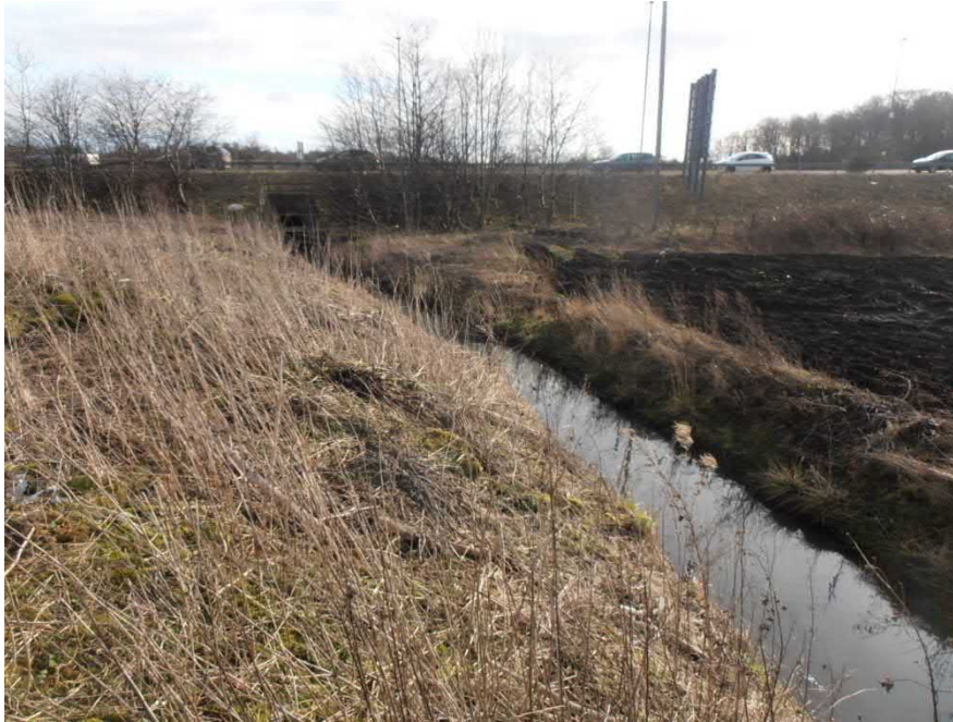
Figure 9 A7 road culvert looking downstream
