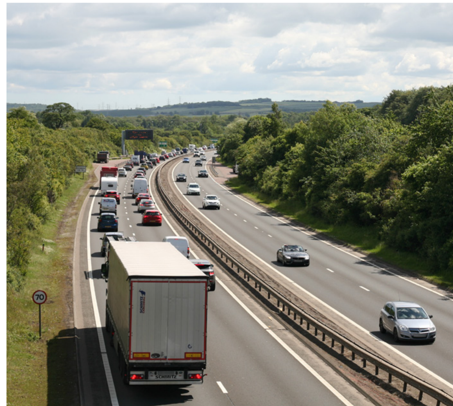
View from the A720 overbridge at Gilmerton junction towards Sheriffhall Roundabout
