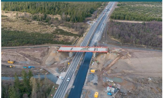
Nine pre-cast concrete beams weighing a total of 390 tonnes were installed during overnight closures of the A9 to create 'The Green Bridge'
