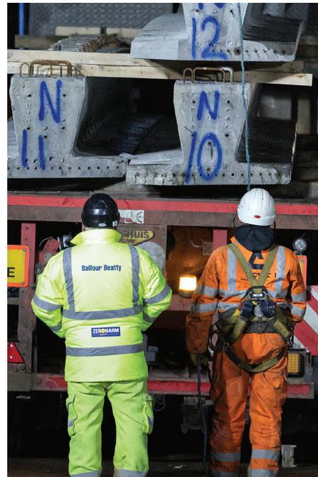
Precast bridge beams being delivered to site ahead of the nightshift to install them
