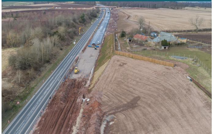
The new line of A9 southbound carriageway takes shape following completion of the soil nail wall to retain the embankment, protecting the neighbouring property
