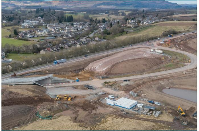
The beam lift operation, which included 23 pre-cast concrete beams, was completed during overnight closures in March 2020 following several weeks of backfill operations
