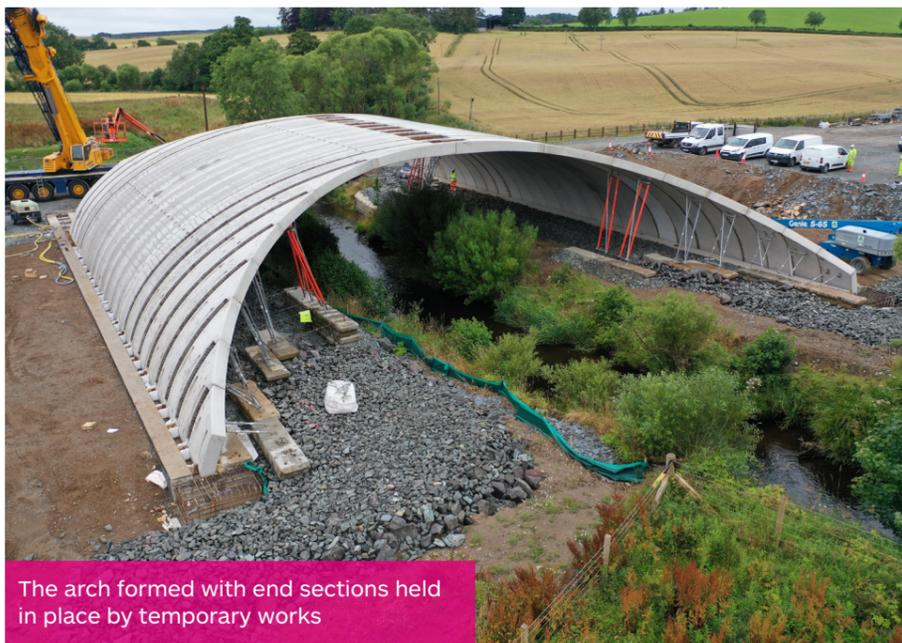
The arch formed with end sections held in place by temporary works
