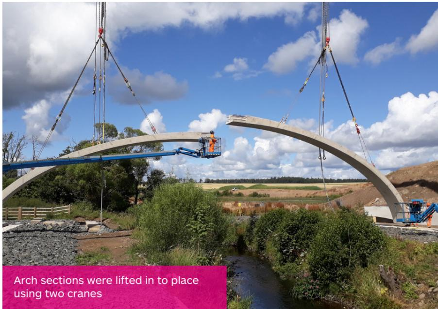
Arch sections were lifted in to place using two cranes
