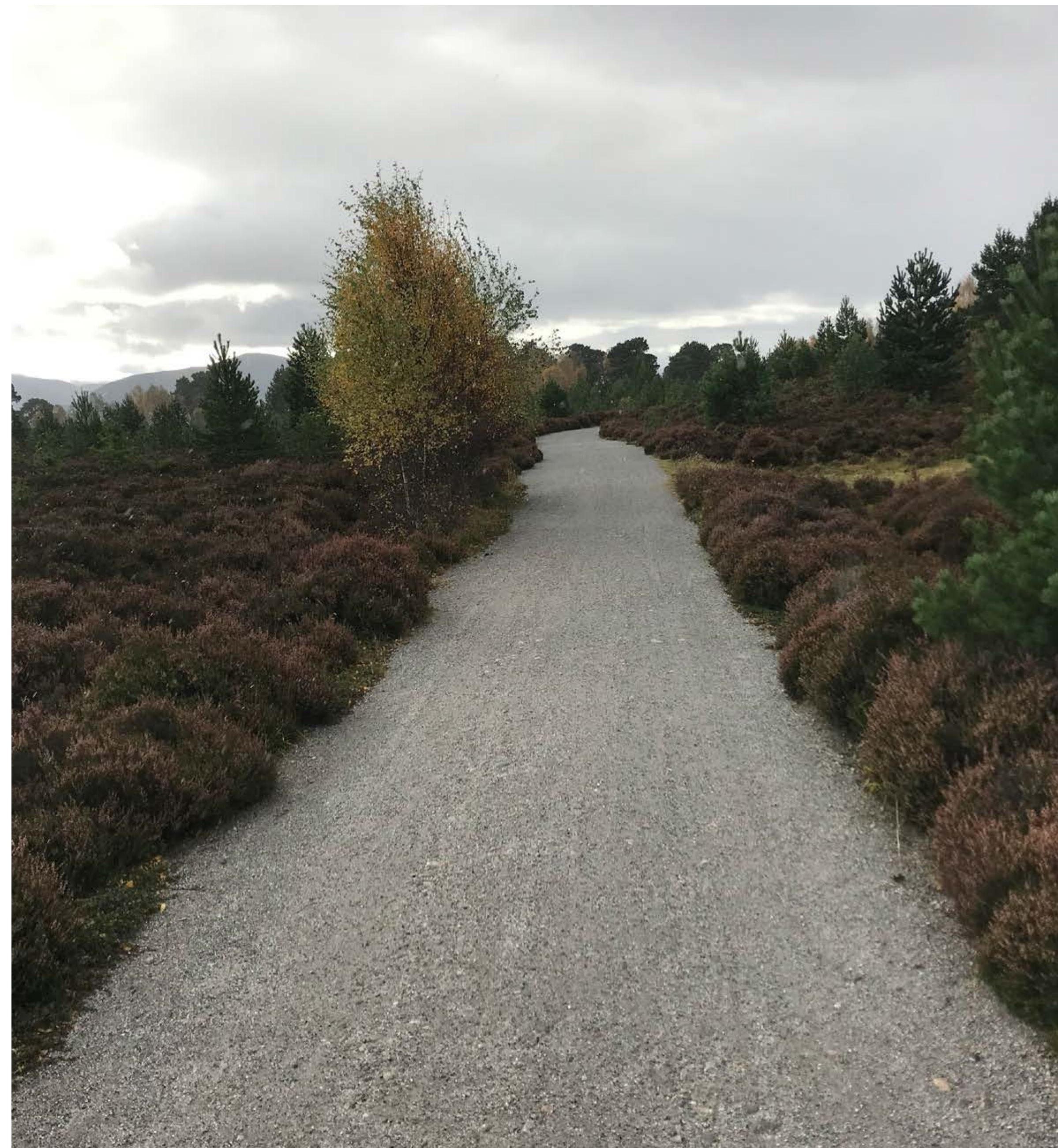
Existing National Cycle Network Route 7 along P2 section to show typical cross section along this route.
