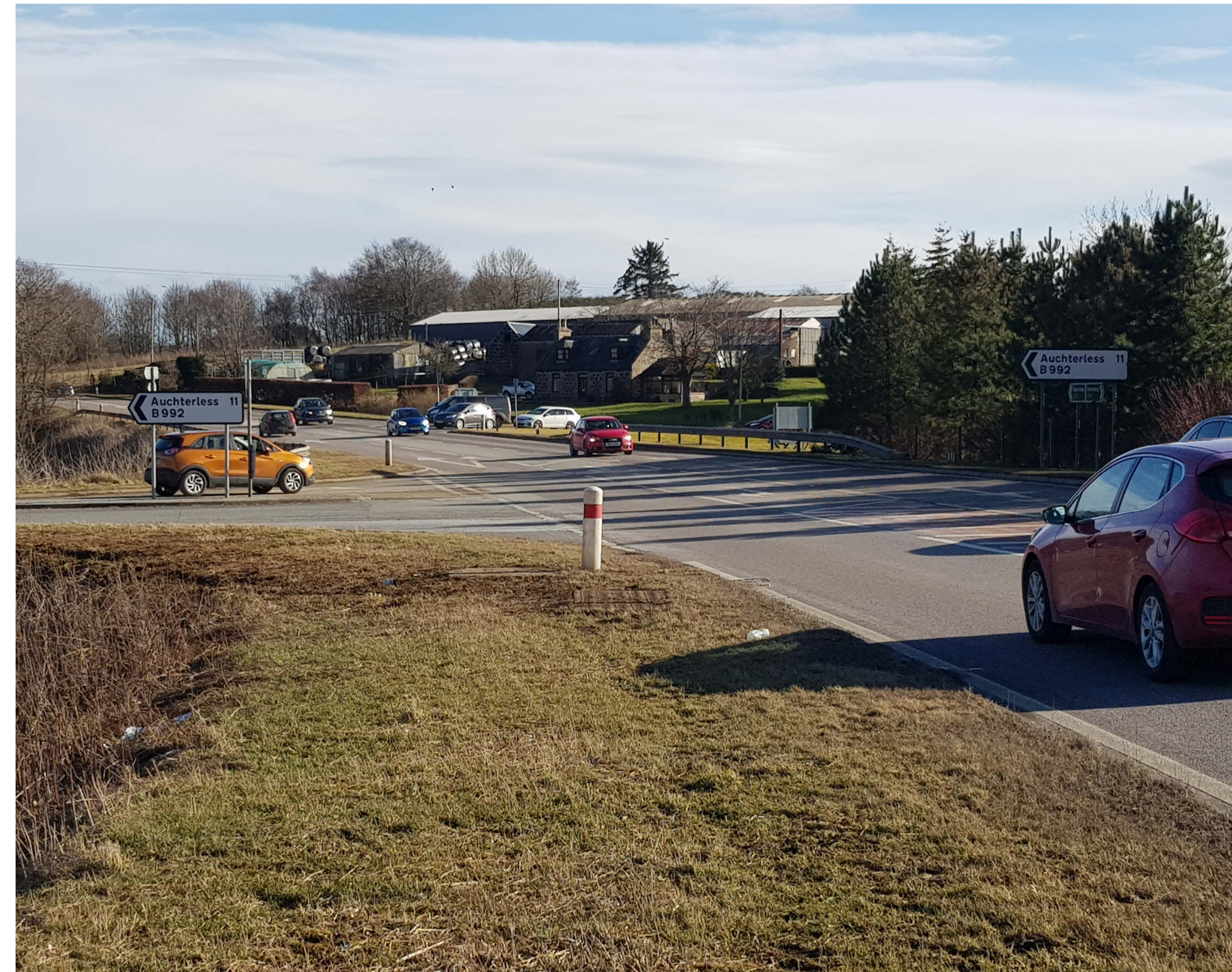
Existing A96 looking east at Kellockbank
