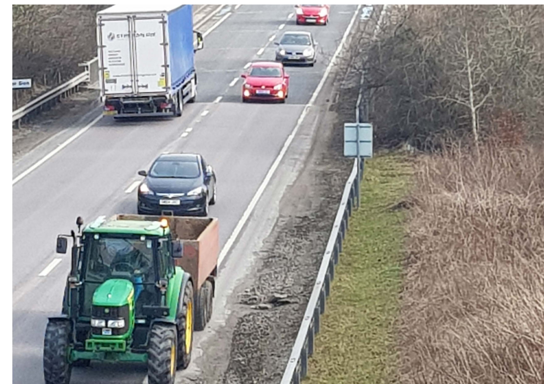
Existing A96 looking east at River Don Crossing
