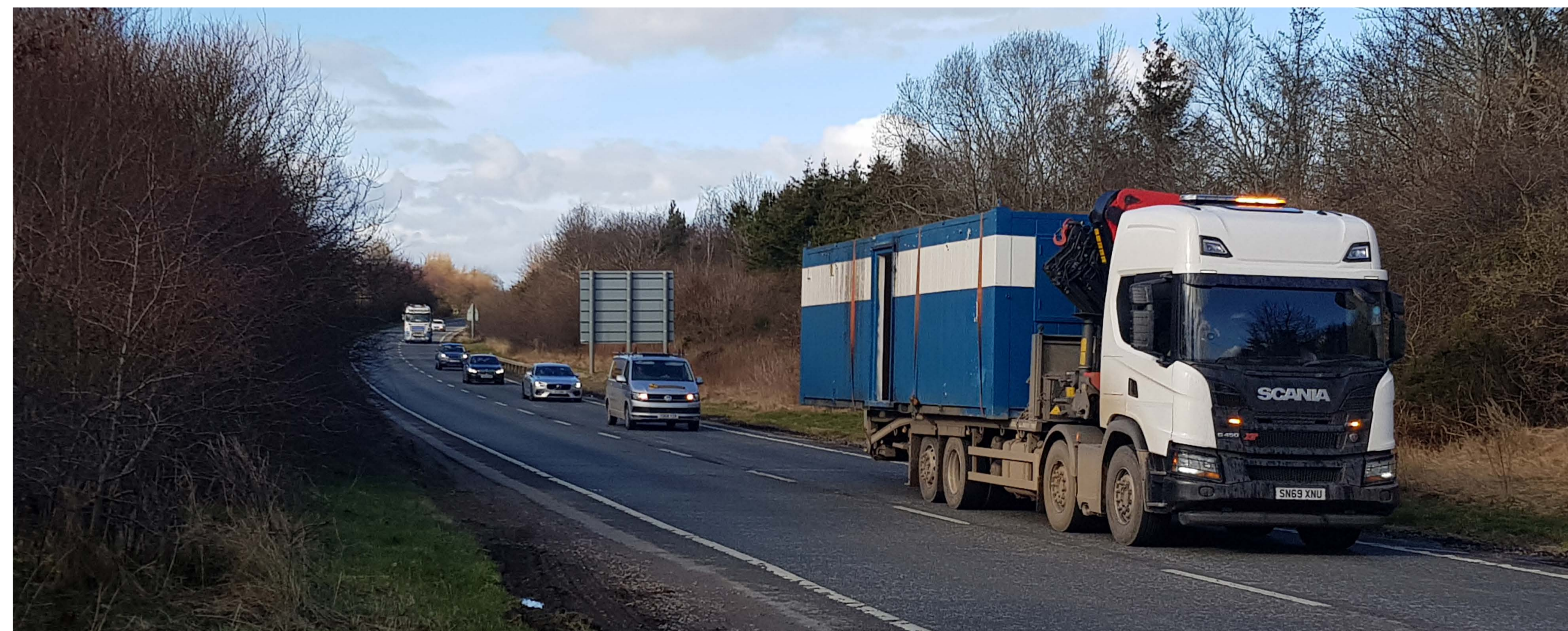
Existing A96 looking west near Blackhall roundabout
