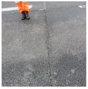
Figure 3.6: Open joint at IP16
