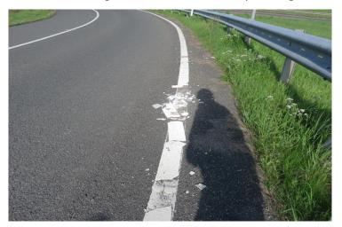
Figure 4.11: Failed road marking
