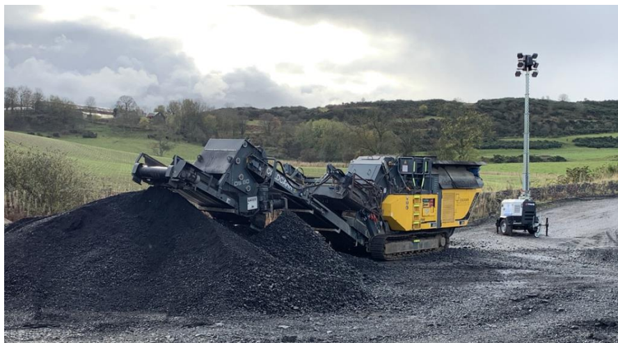
Figure 2-3 - Crushing and screening of arisings (courtesy of BEAR NE)
