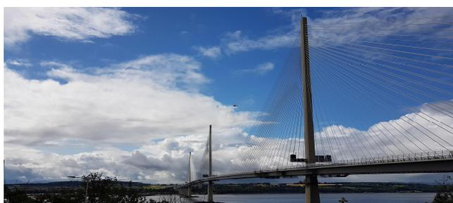
Figure 18: Queensferry Crossing – 3 tower cable stayed bridge
