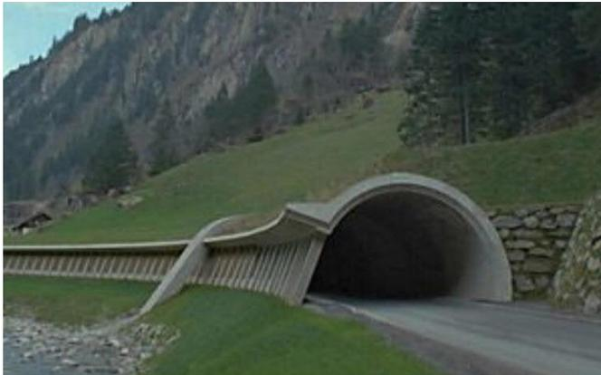
Figure 4: Example of a Debris Shelter to Protect Road from Rockfall
