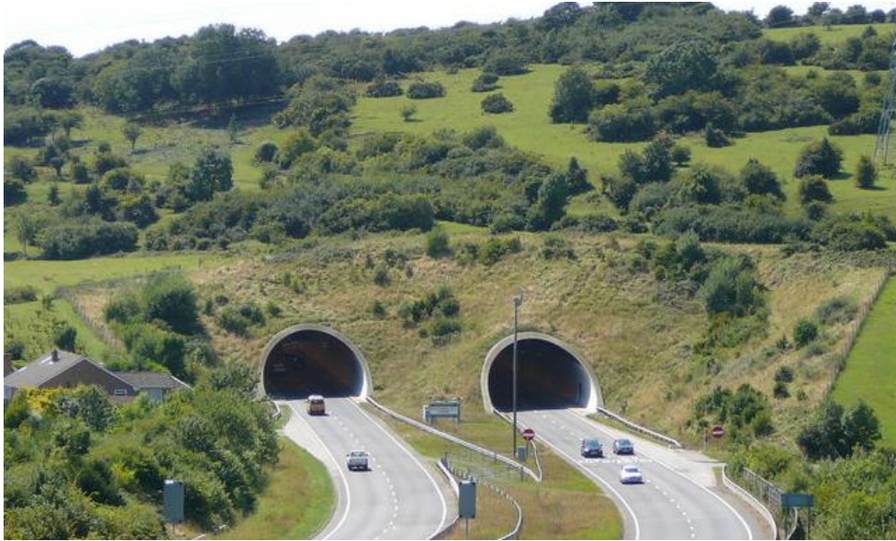
Image C9.31: Example of a tunnel portal with low visual 'clutter' - A27 Southwick Hill Tunnels / © Colin Park / cc-by-sa/2.0
