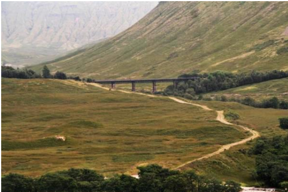
Image C9.28: Example of a simple viaduct structure - Railway viaduct over Allt Coralan, on the "Horseshoe" / © Chris / cc-by-sa / 2.0
