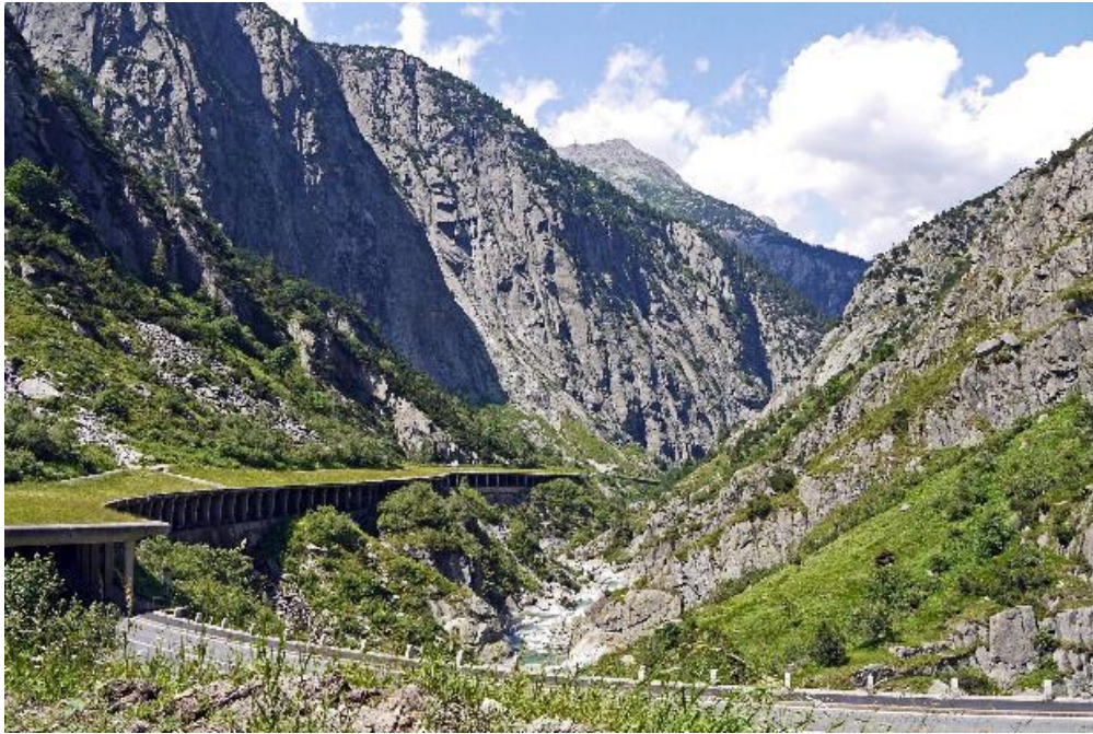
Image C9.22: Example avalanche protection gallery in Gotthard Pass, Switzerland © Erich Westendarp via Pixabay
