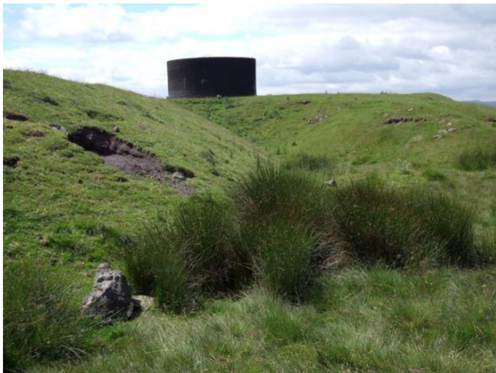
Image C9.35: Example of a tunnel ventilation shaft - Totley Tunnel ventilation shaft, Diggle / © Stephen Burton / cc-by-sa/2.0
