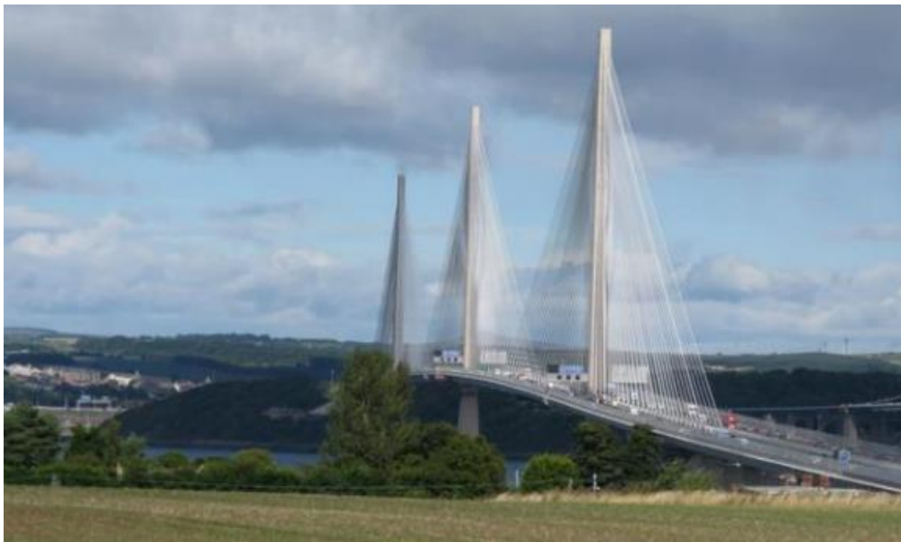
Image C9.26: Example of a large-scale elegant placemaking structure - Queensferry Crossing / © G Laird / cc-by-sa/2.0
