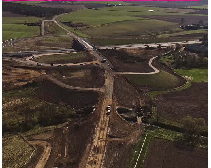
U32 Tullybelton Road looking east, April 2021
