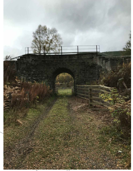
Pedestrian underpass under rail embankment
