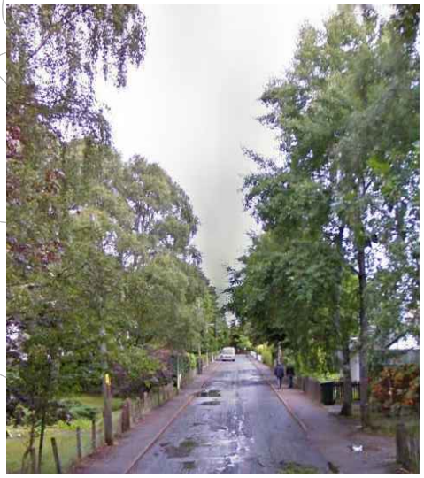
Kinchurdy Road/NCN7/LBS116. Footways adjacent to property frontage and accesses.
