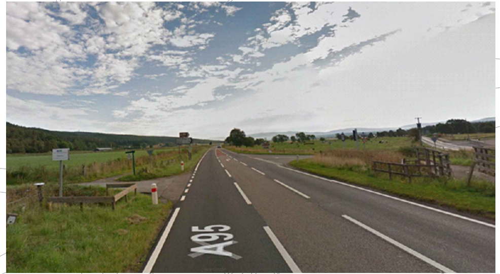
Formal uncontrolled crossing from Deshar Road/ NCN7 to Core Path LBS53.
