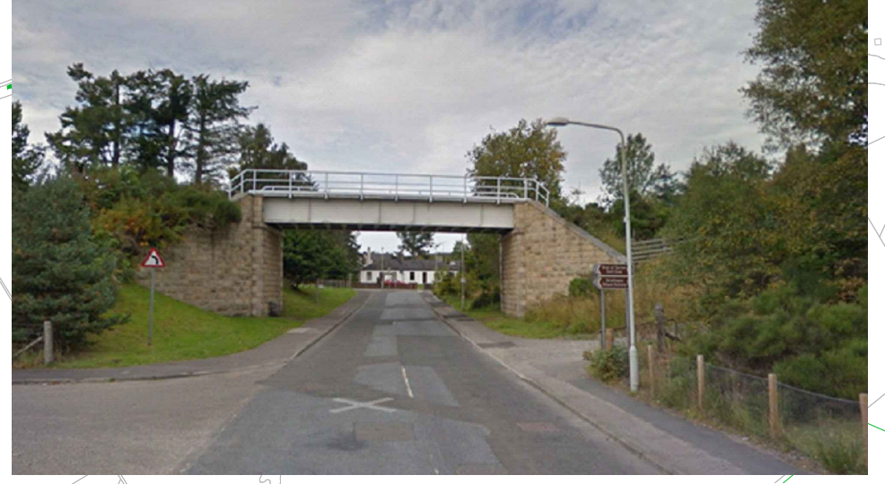
Railway line overbridge.
