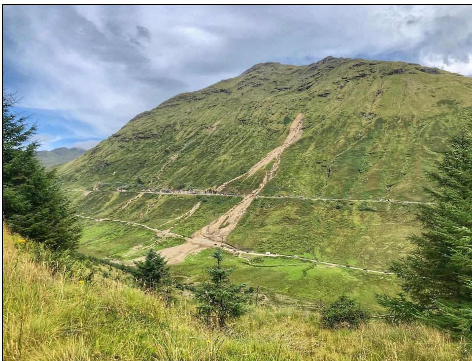
Figure 1.1: Photo Of The A83 Road And Landslide Taken August 2020.
