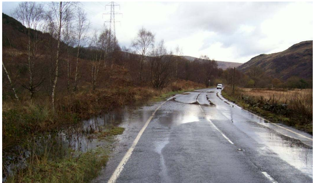
Photo 2.5: Flooding of the A82 at Garabal
