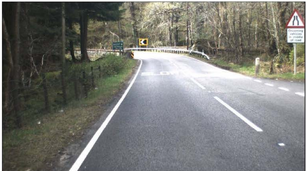
Photo 2.3: A82 southbound approaching Inveruglas Water bridge
