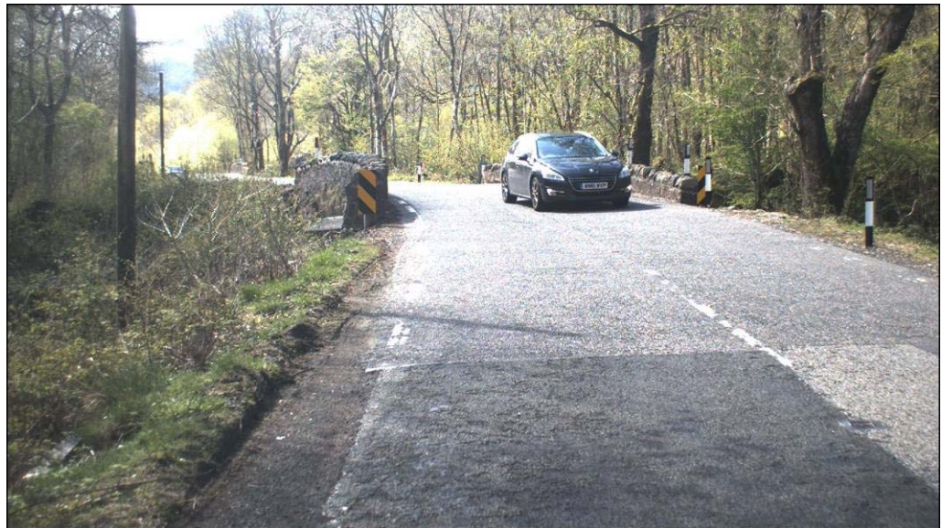
Photo 2.4: Width restriction of existing bridge south of Inverarnan
