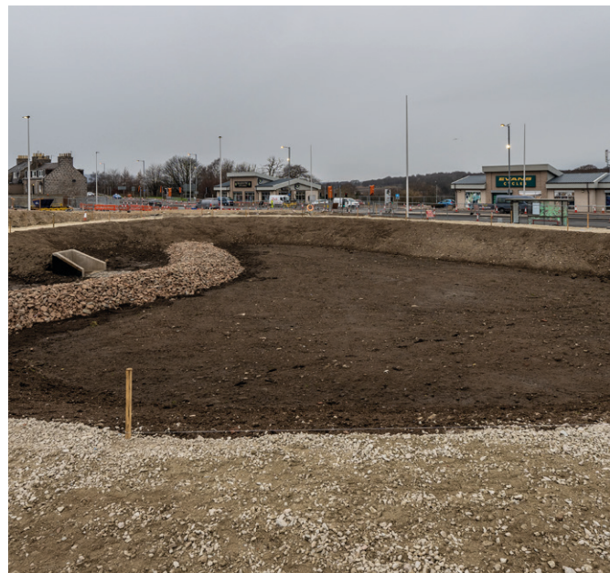
Formation of the Sustainable Drainage System (SuDS) basin
