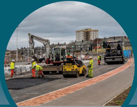
Surfacing work on new link road
