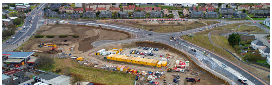
Overview of the new dual carriageway link road.
