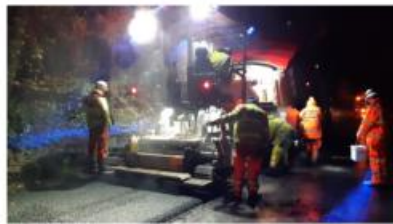
A82 North of Pulpit Rock - Resurfacing
