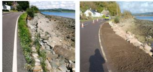
A83 Ardrishaig - Coastal Protection (before and after)
