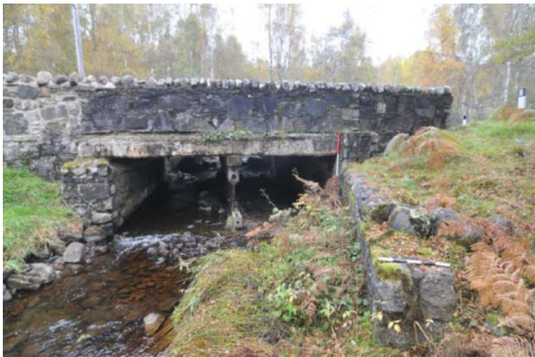
Figure 1 - Allt Lagain Bhain Bridge
