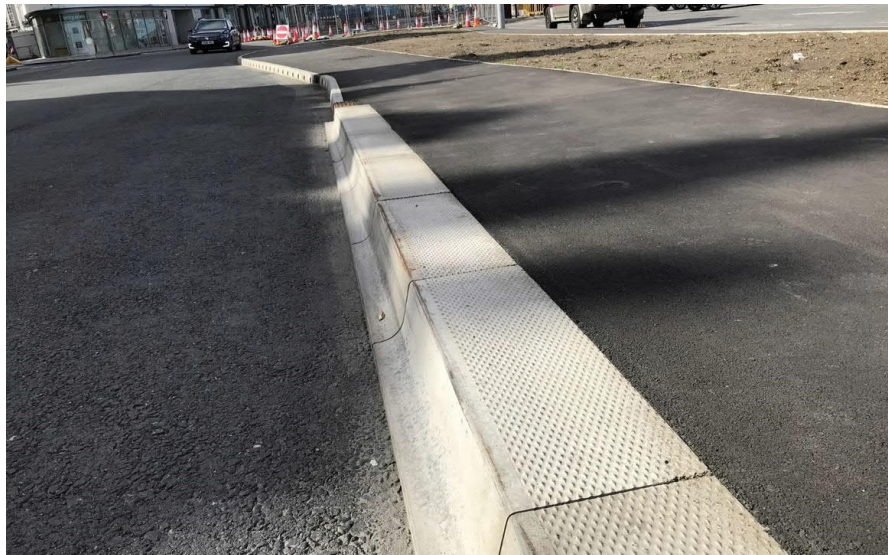
Figure A.2: Kassel Kerb
