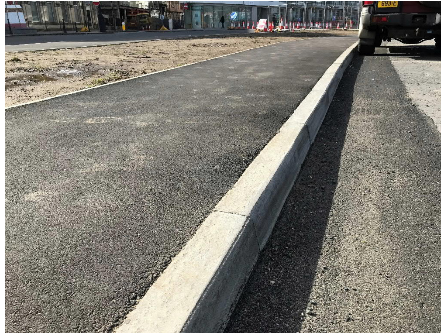
Figure A.21: Square kerb at construction site
