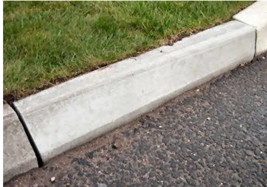
Figure A.25: Splayed to Half-battered Transition kerb
