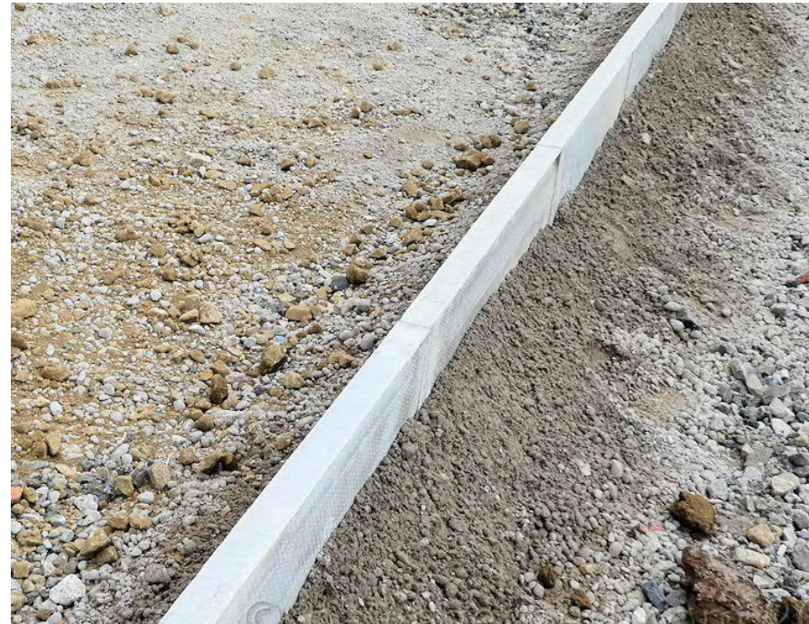
Figure A.13: Type EF Edging kerb under construction
