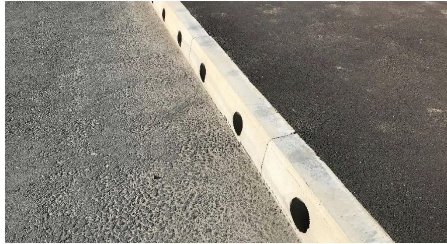
Figure A.17: In-situ drainage kerb
