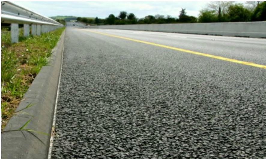
Figure A.22: Splay kerb on high speed road
