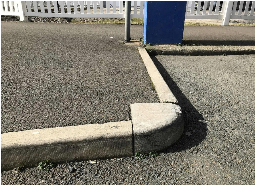
Figure A.18: Quadrant kerb
