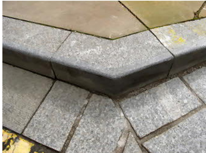
Figure A.19: Angle kerb
