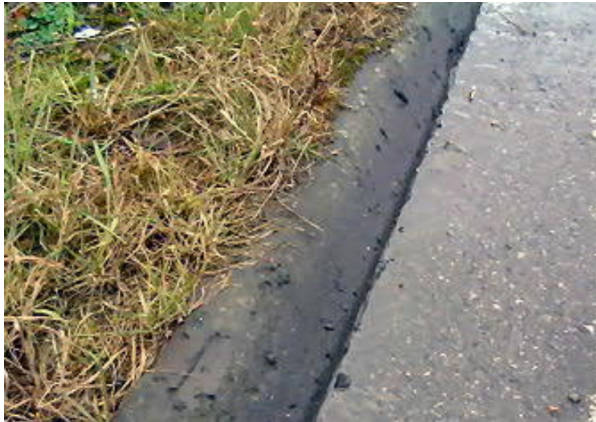
Figure A.14: Extruded asphalt kerb on UK Motorway
