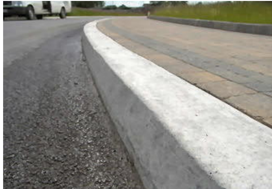
Figure A.15: Slip-formed concrete kerb on Irish housing estate
