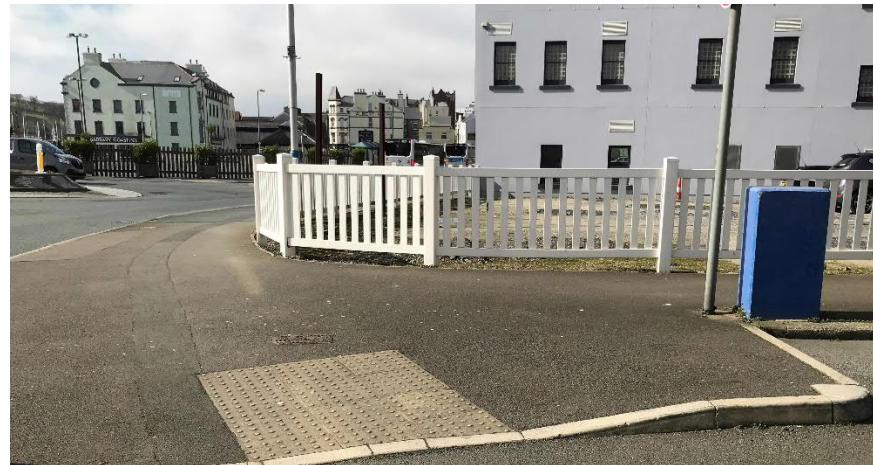
Figure A.11: In-situ dropped kerb
