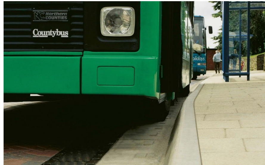
Figure A.3: Marshalls Bus Stop Kerb
