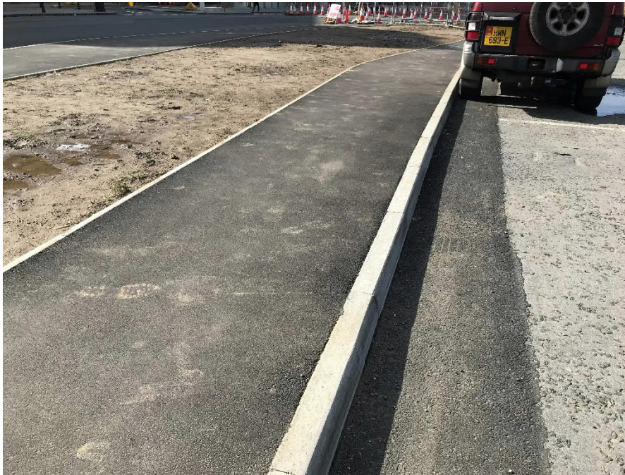
Figure A.20: Square kerb at construction site
