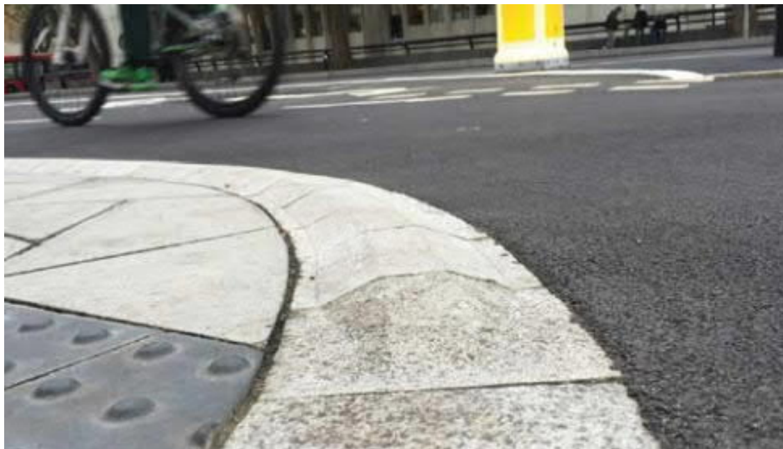
Figure 3.5: Trapezoidal edge strip detail
