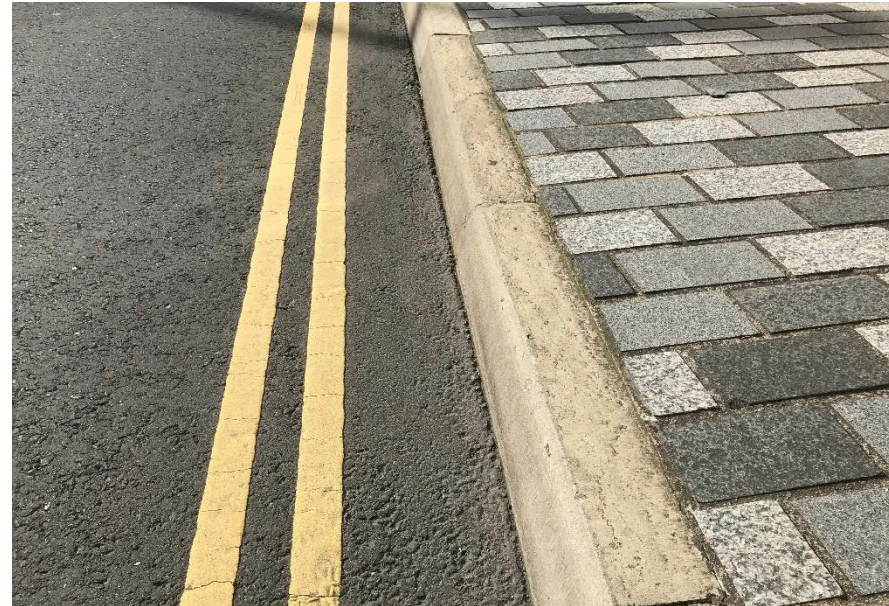
Figure A.5: In-situ Half-battered kerb
