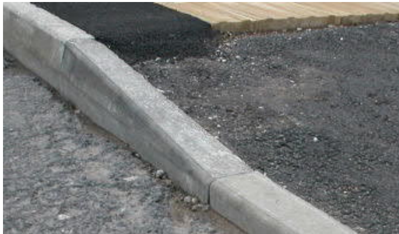
Figure A.10: Dropped kerb at crossing point under construction
