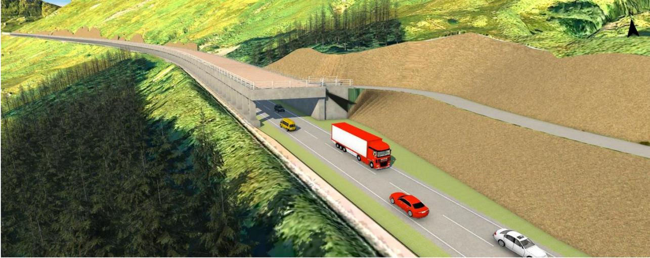
**Figure 5-17 - Visualisation of the southern entrance to the Brown Option Debris Flow Shelter, looking north up Glen Croe**
