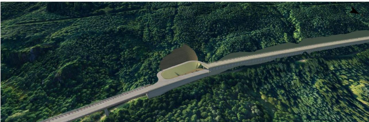
**Figure 5-28 - Visualisation of the southern maintenance access from the proposed A83 to the roof of the Green Option debris flow shelter**
