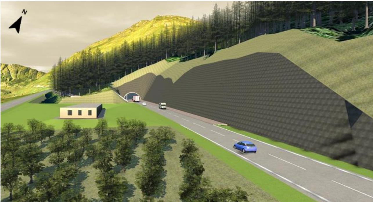
**Figure 3-11 - Visualisation of the southern entrance to the Pink Option tunnel and the temporary diversion of the A83.**
