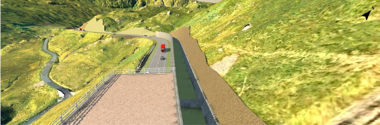
**Figure 5-15 - Visualisation of the Brown Option Debris Flow Protection Wall looking north up Glen Croe**
