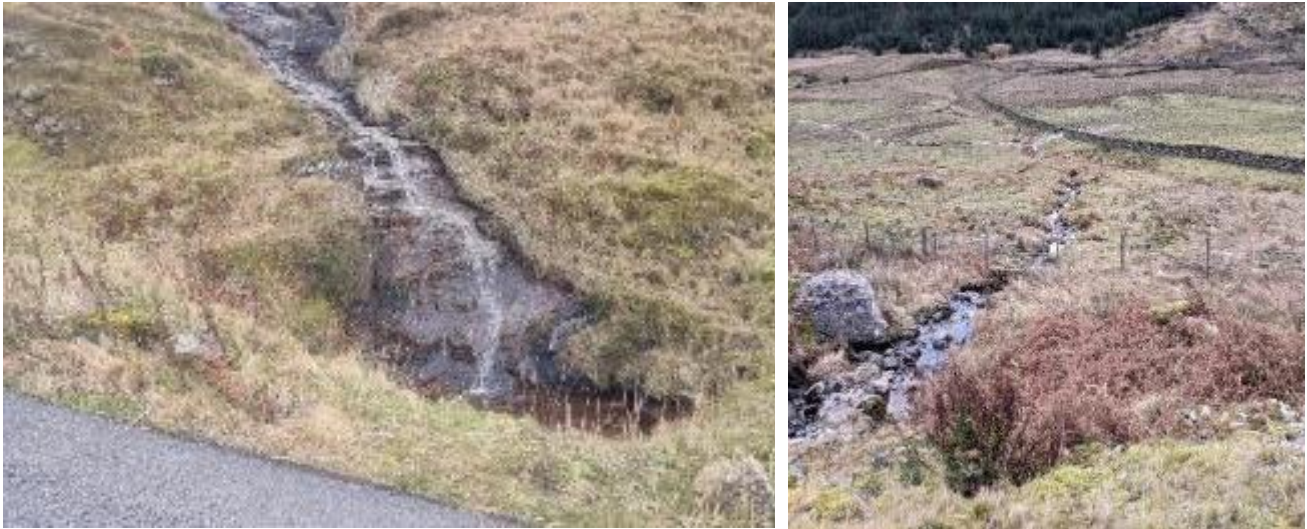
Plate 15.8 Typical channels along the OMR route (Dated: 09 December 2022)
